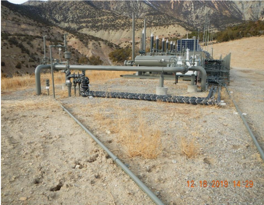
Dead weed debris around heated separators.
