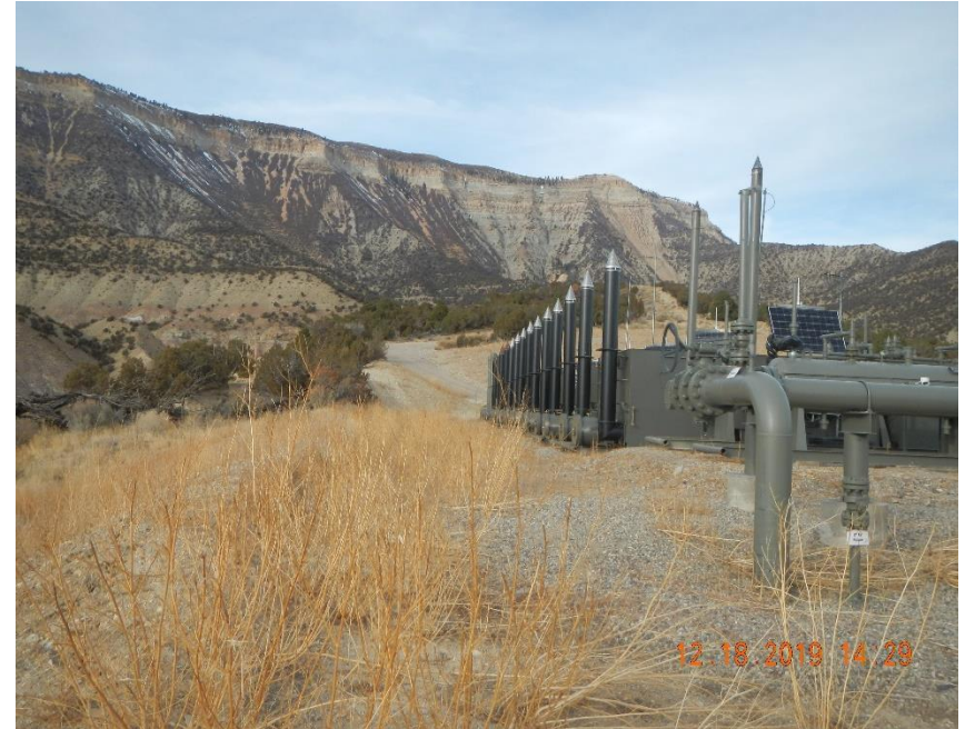
Dead weed debris around heated separators.
