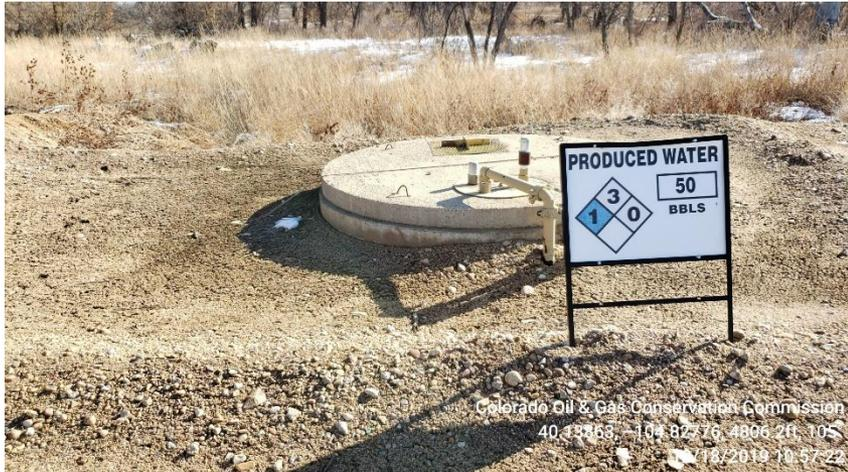
**Photo 7 Produced water Berm inadequate**
