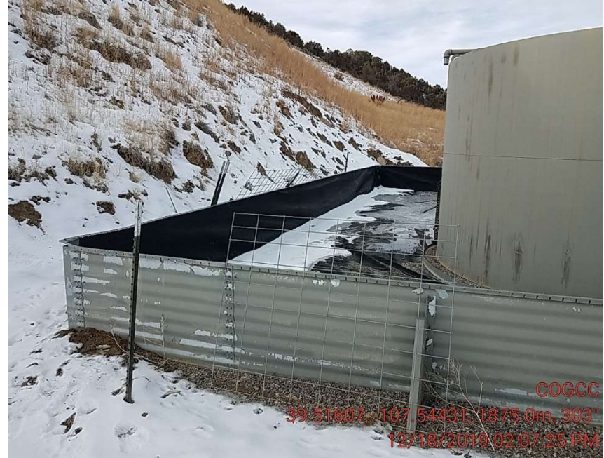
Fencing not installed
