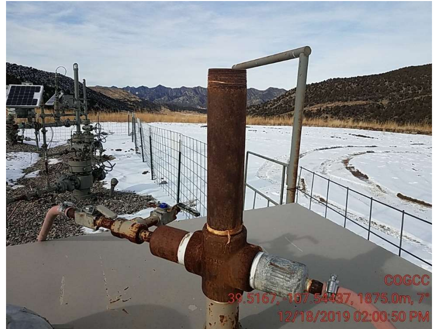
Pipe is open to atmosphere
