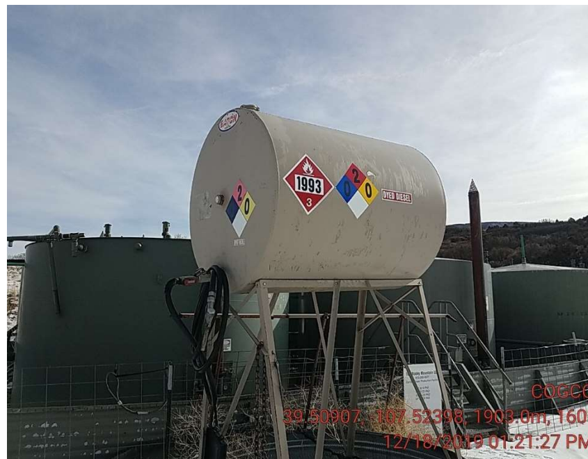
Missing tank information on fuel barrel. No capacity, or operator.
