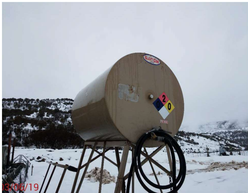
Missing tank information on fuel barrel. Photo from previous inspection.
