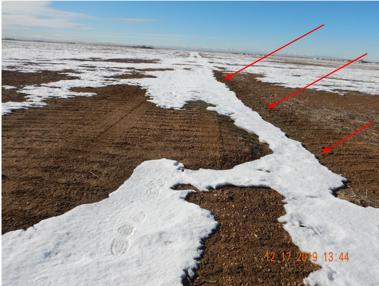
Photo 2. Photo taken from the eastern access road, facing West. Photo illustrates access road has not been contoured to match the surrounding landscape.
