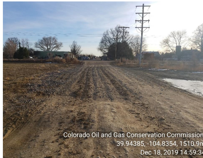
Photo 2 rock tracking pad impacted with sediment.
