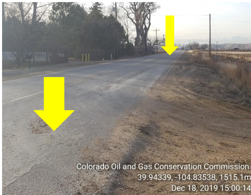
Photo 3 Sediment being carried off right away on to county road
