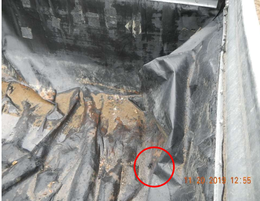
Photo #9 - View of the 1-inch hole on the northeast corner of the tank battery (Red circle).
