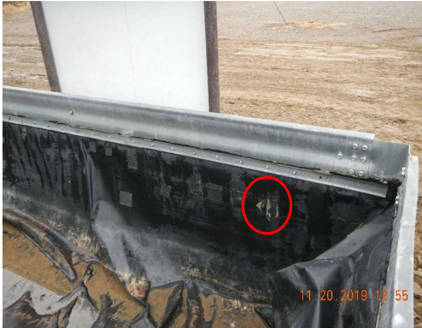
Photo #13 – View of the patches missing on the northeast corner of the tank battery secondary containment (Red circle).
