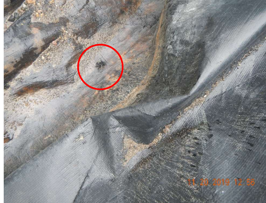
Photo #8 – View of the 1-inch hole on the northeast corner of the tank battery (Red circle).
