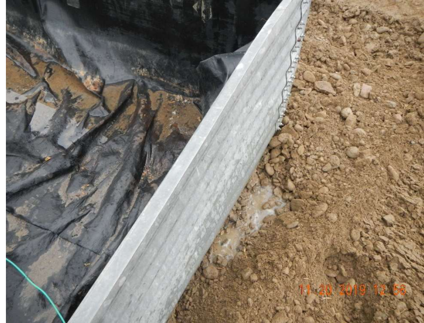
Photo #10 – View of fluids daylighting outside of the secondary containment adjacent to the observed 1-inch hole in the liner.
