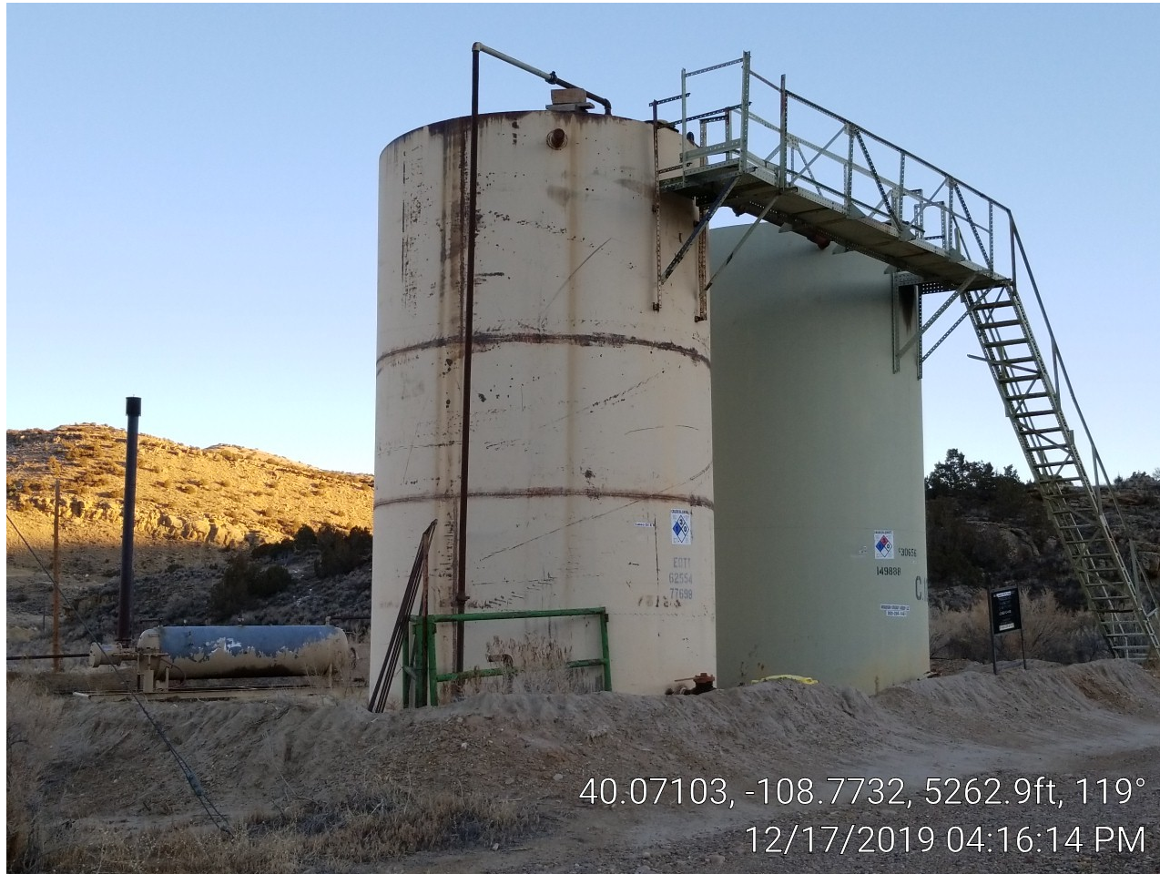
Photo 2. Tank battery.
