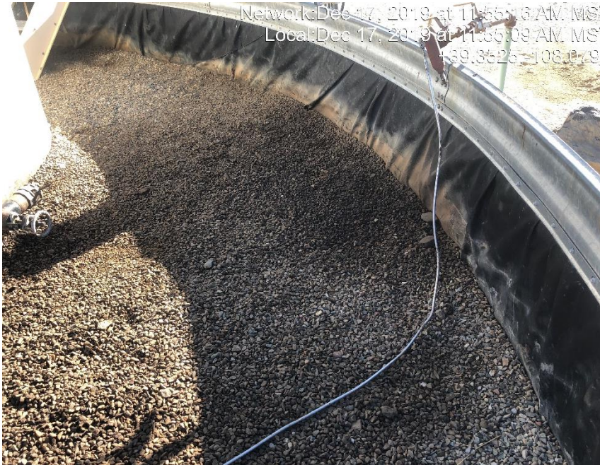
Photo #0268 stained gravel inside tank containment.
