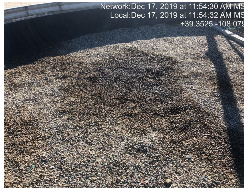
Photo #0267 stained gravel inside tank containment.
