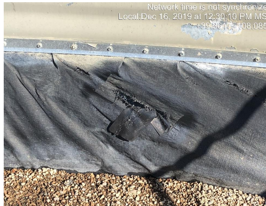
Photo #0261 Multiple holes in tank containment liner.
