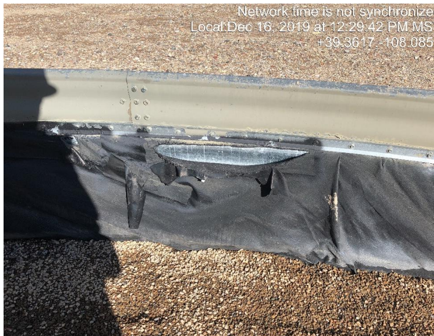
Photo #0260 Multiple holes in tank containment liner.
