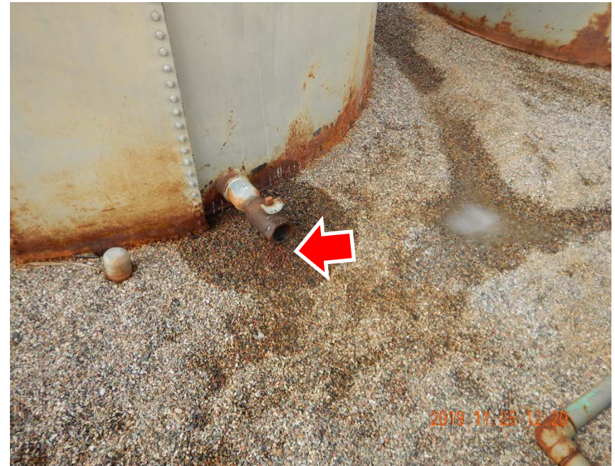
Photo #12 – Unidentified fluids observed in threads and rust-stained gravel beneath ball valve attached to tank in NE corner of containment area (1).
