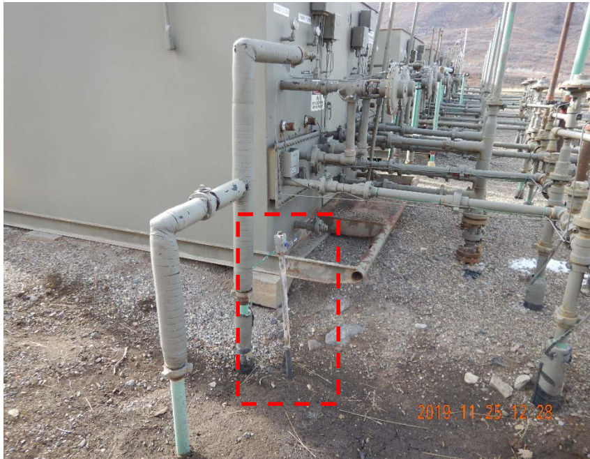
Photo #11 – Capped, unmarked 1" flowline riser located east of separators.
