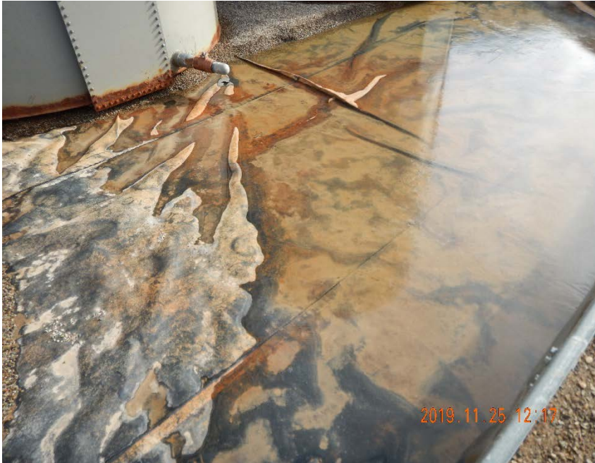
Photo #3 – Gravel base has been removed from southwest corner of tank battery in response to Spill/Release ID #467054.
