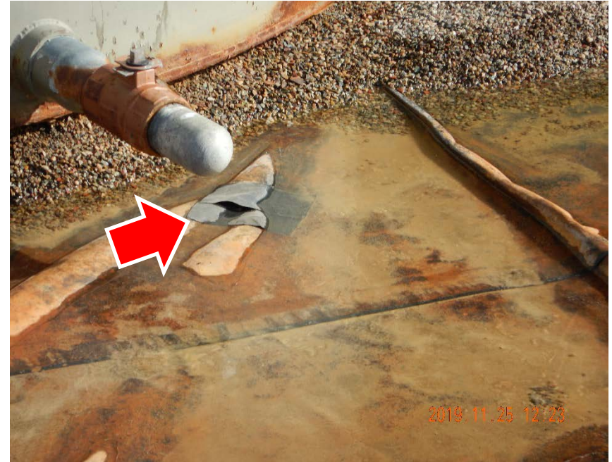
Photo #4 – Patched area of tank battery liner had an apparent gap during inspection. Operator was notified of issue via phone on 11/26/2019.
