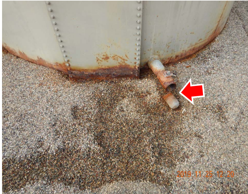
Photo #13 - Unidentified fluids observed in threads and rust-stained gravel beneath ball valve attached to tank in NE corner of containment area (2).
