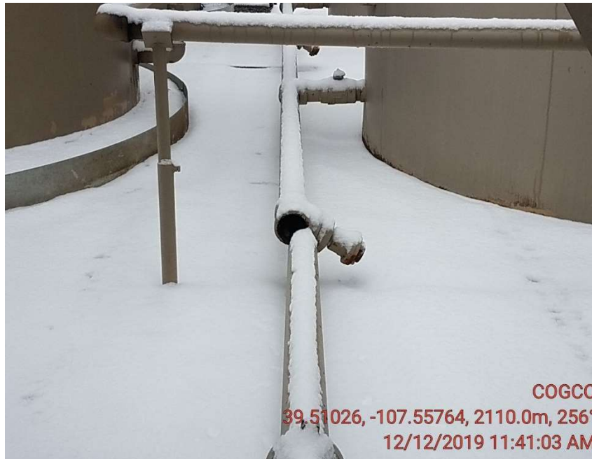
PIPEING NOT CONNECTED
