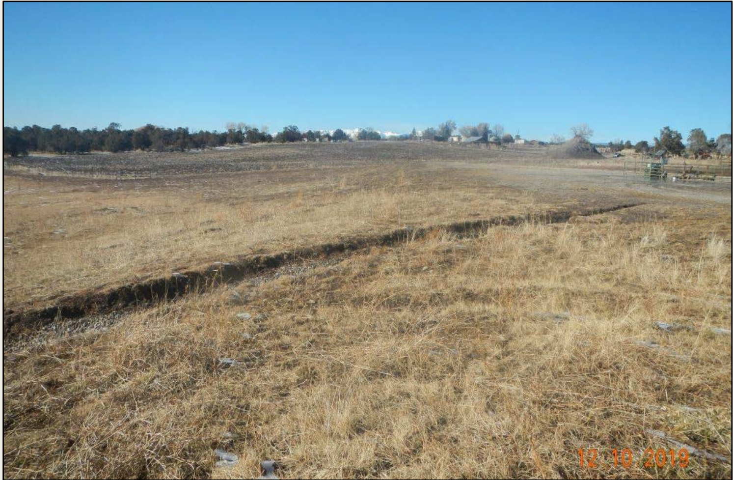
Photo 3. View of the southwestern fill slope from the southern corner facing northwestward. Revegetation appears to be progressing, in a dormant and grazed condition with grasses such as western wheat grass and sand dropseed.
