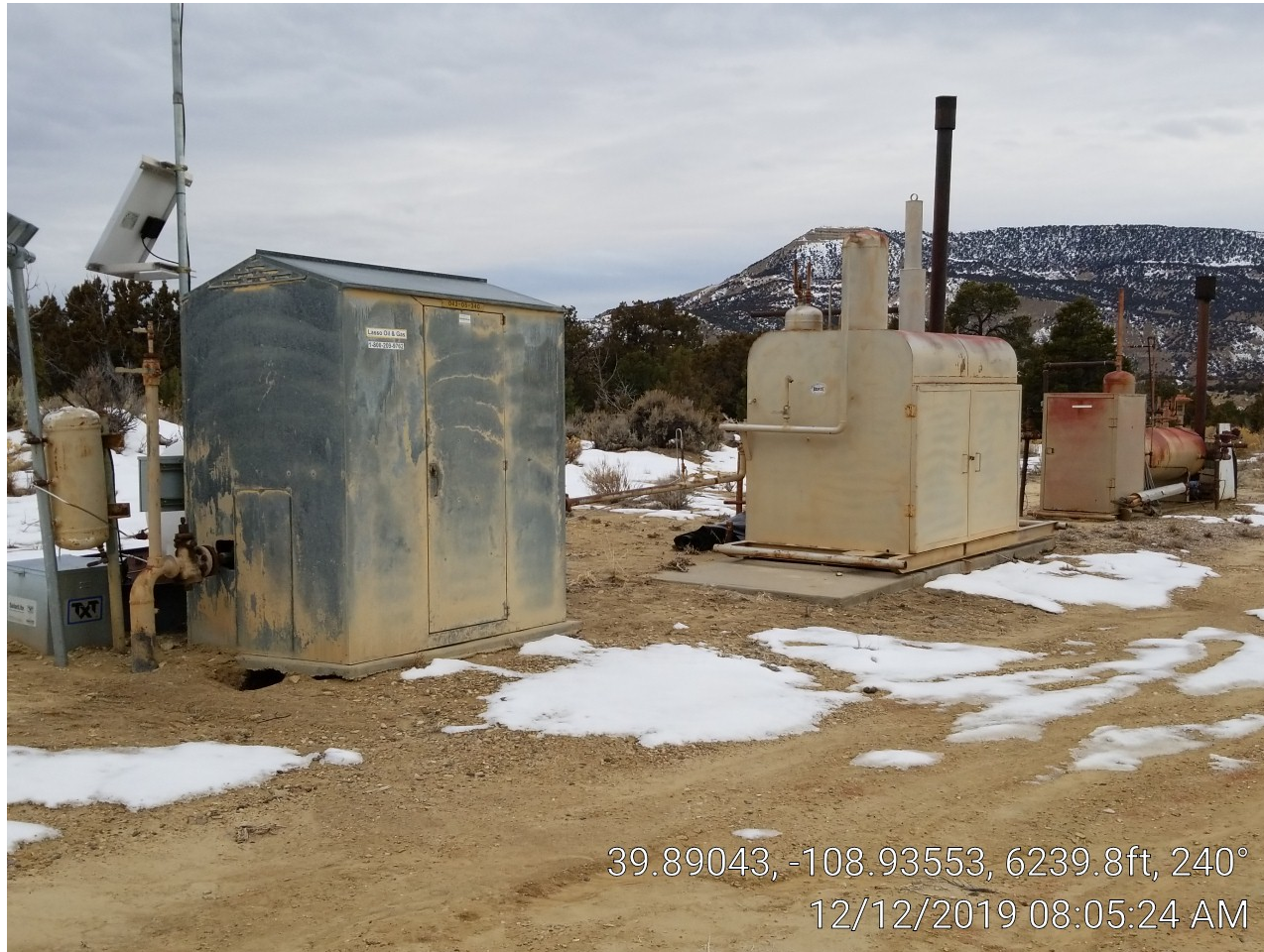
Photo 3. Meter building & separators.
