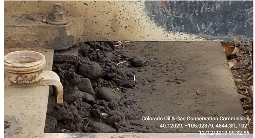
**Photo 3 Stained soil by gas engine exhaust**
