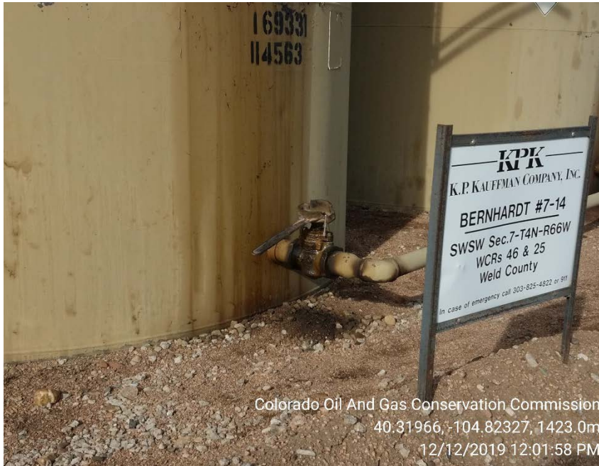
Load valve and stained soil
