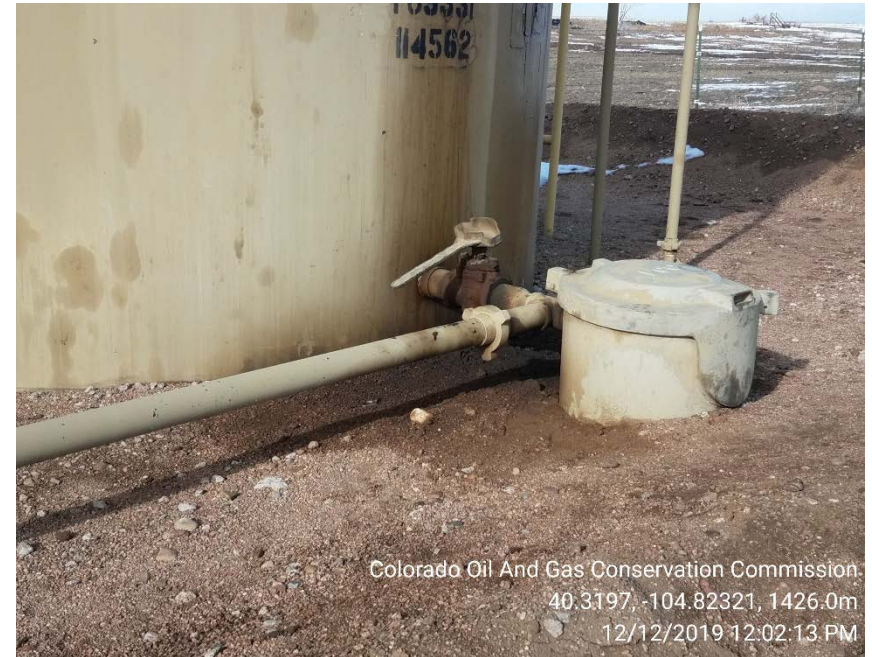
Load valve and stained soil
