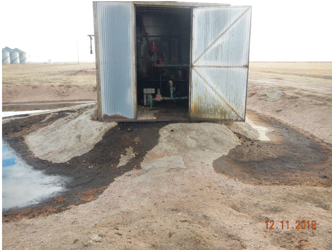
Photo # 6 – Oil spill within treater berm
