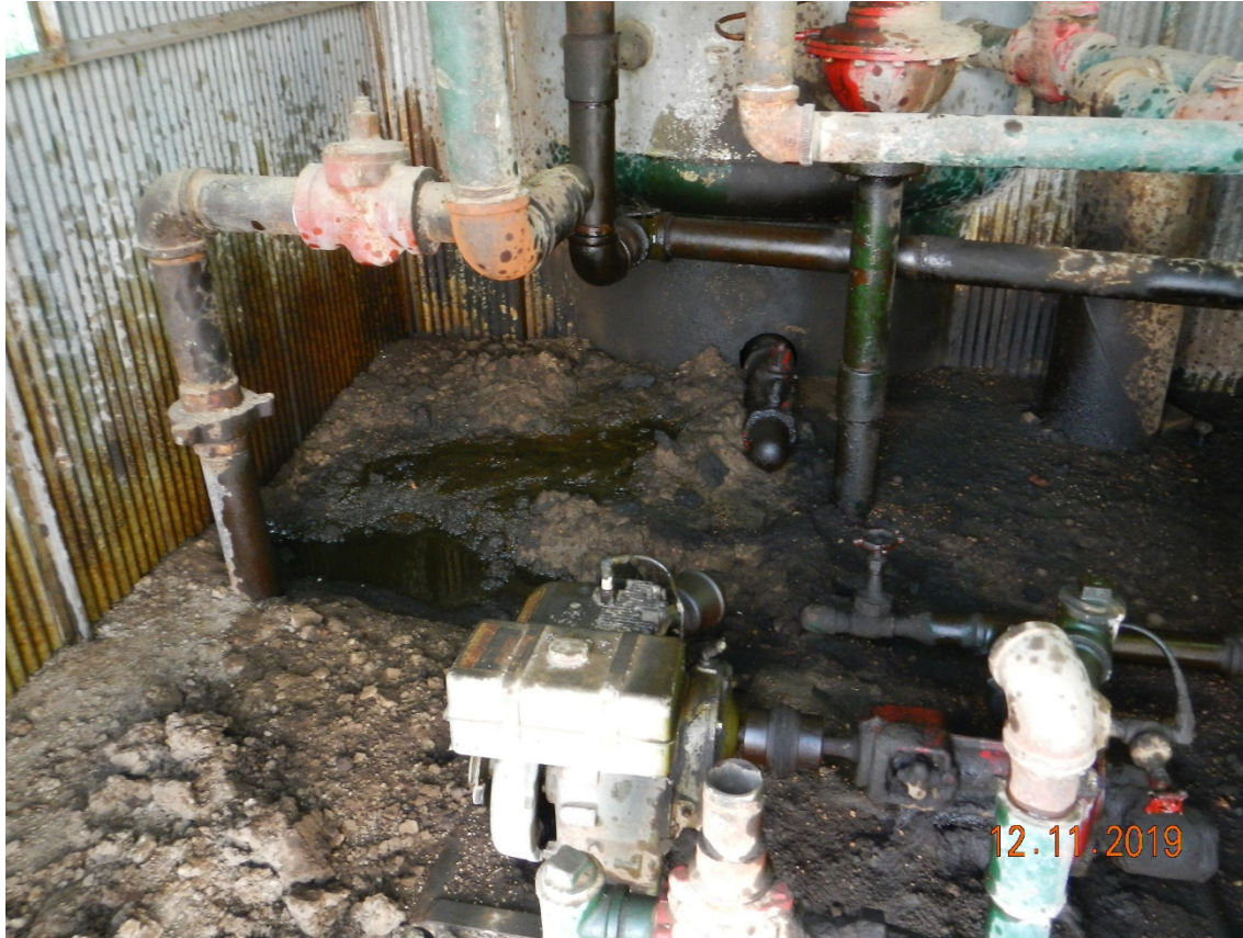
Photo # 7 – Oil spill within treater berm
