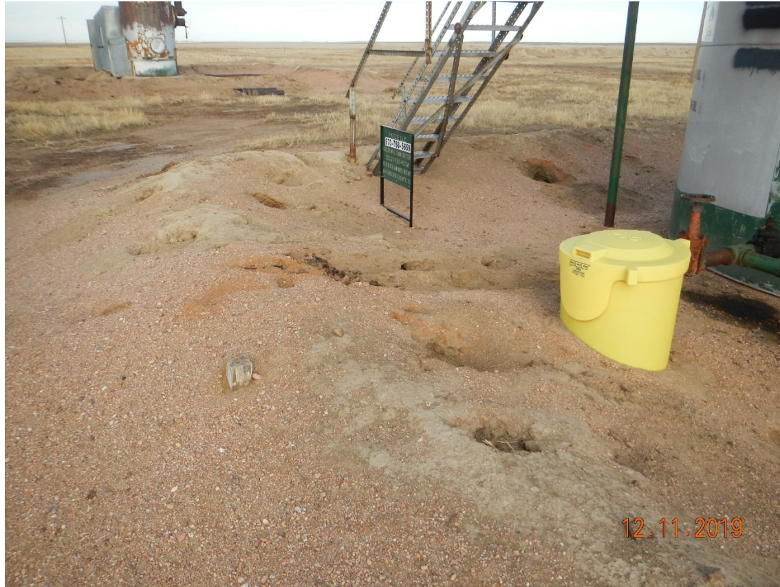
Photo # 3 – Animal burrows in tank battery berm
