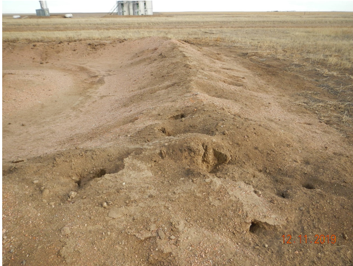
Photo # 4 – Animal burrows in tank battery berm
