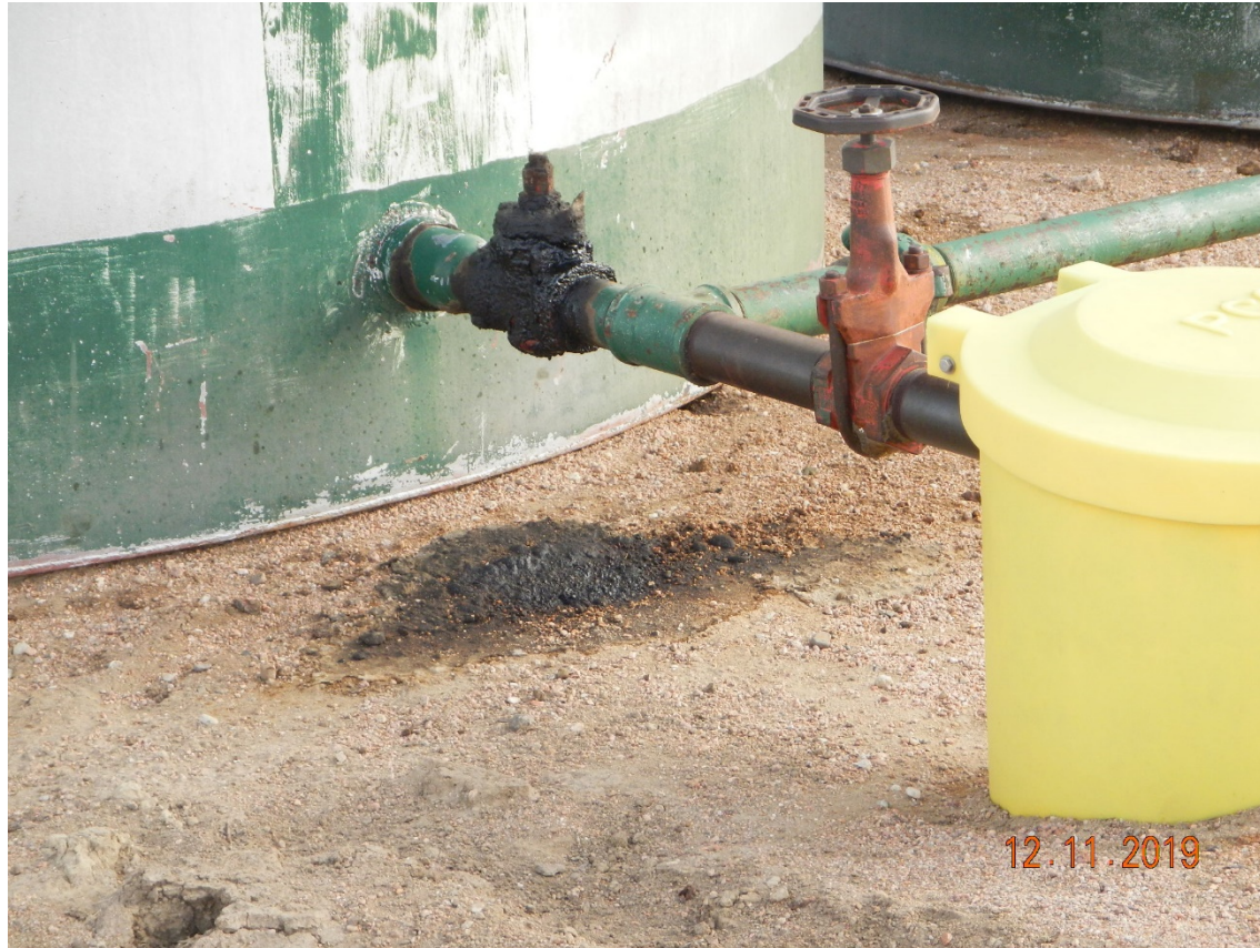
Photo # 2 – Minor oil staining at crude tank loadout area
