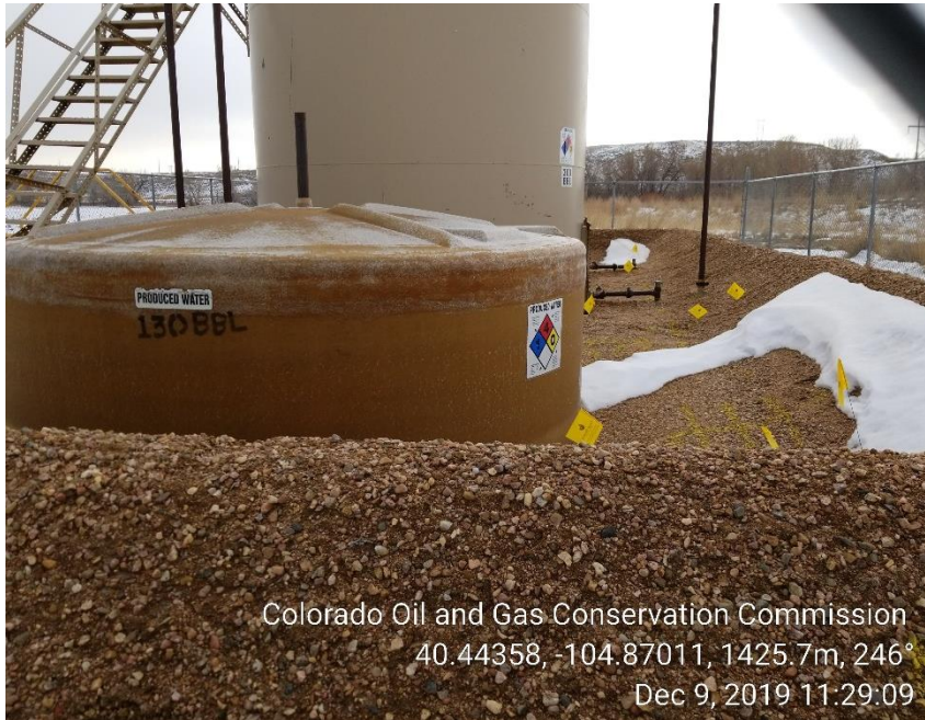
Photo 3: H2O tank not anchored
