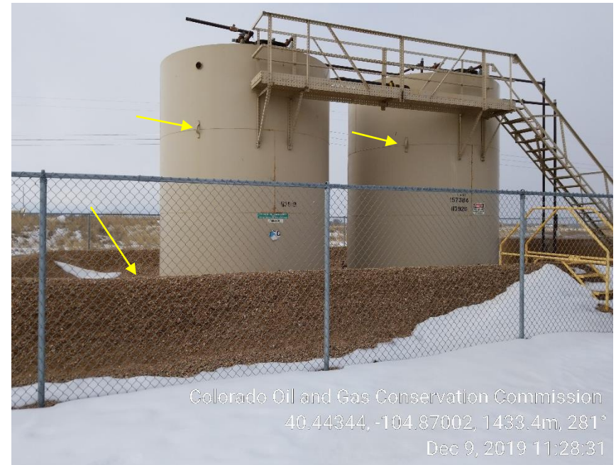
Photo 2: Tank Battery; inadequate berm/tanks not anchored
