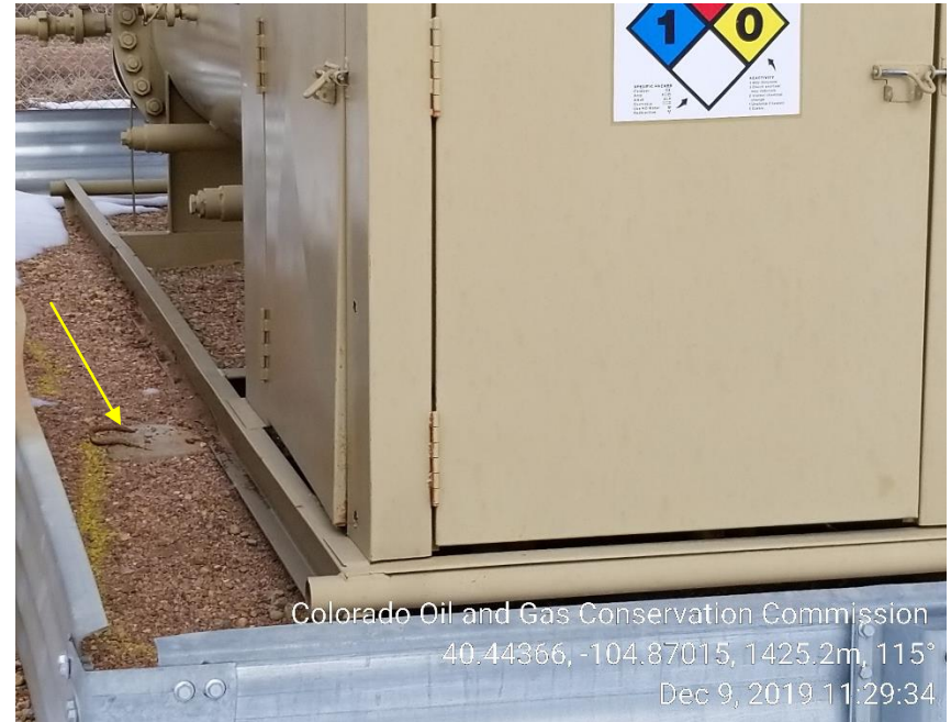
Photo 4: Separator not anchored
