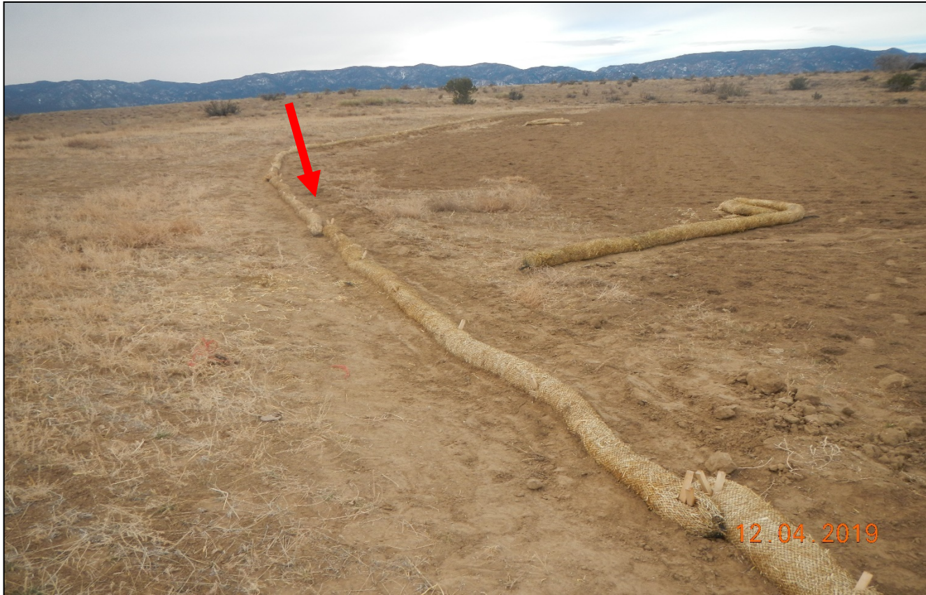
Photo 4. Facing west toward the southern portion of the location. A berm, small ditch, and wattles are installed around the southern perimeter. The concern is that the ditch is directed downhill which can accelerate stormwater and cause erosion.
