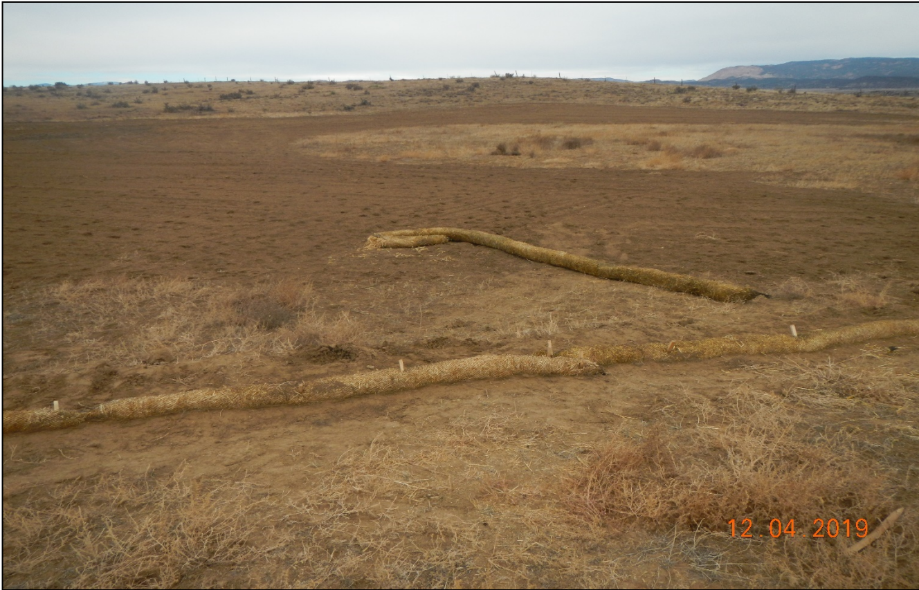
Photo 3. Facing northwest toward the location. There are wattles displaced at the southeast side.
