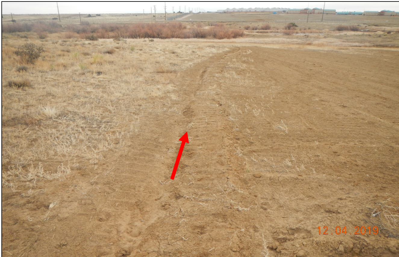
Photo 8. Facing east toward the northern portion of the location. A berm and small ditch are installed around the southern perimeter. The concern is that the ditch is directed downhill which can accelerate stormwater and cause erosion.
