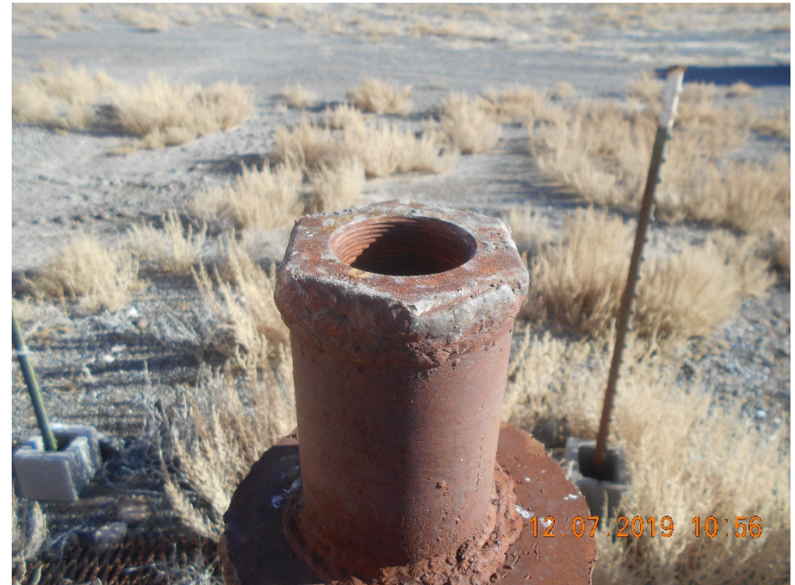
Open ended production casing.
