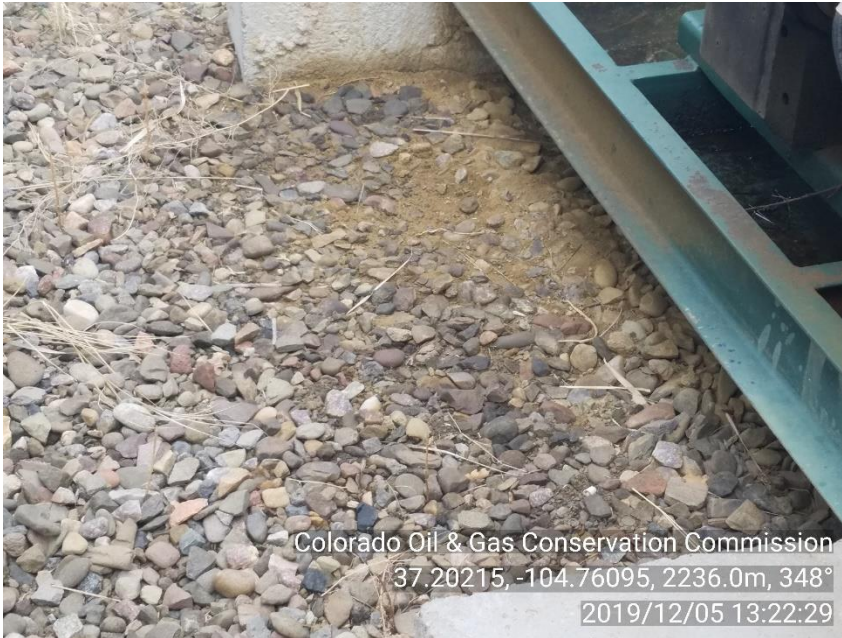
PHOTO 5: OILY IMPACTED SOIL NEAR ENGINE SKID. Remove and dispose impacted material in approved manner, service and maintain equipment and self inspect to prevent recurrence of conditions per 1002.f(2) and 907. CA DATE 01-05-20
