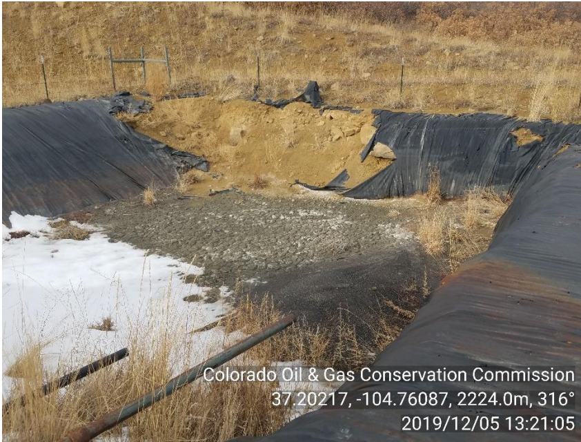
PHOTO 3: LINER HAS DETERIORATED AND HAS SEVERAL HOLES IN IT. REMOVE (IF NOT REQUIRED) OR MAINTAIN LINER IN ACCORDANCE WITH RULE 904. CA DATE 02-05-20
