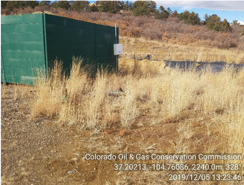
PHOTO 9: GRASS/WEEDS AROUND WELLHEAD. CUT/MAINTAIN GRASS/WEEDS IN ACCORDANCE WITH RULE 603.f. CA DATE 01-05-20
