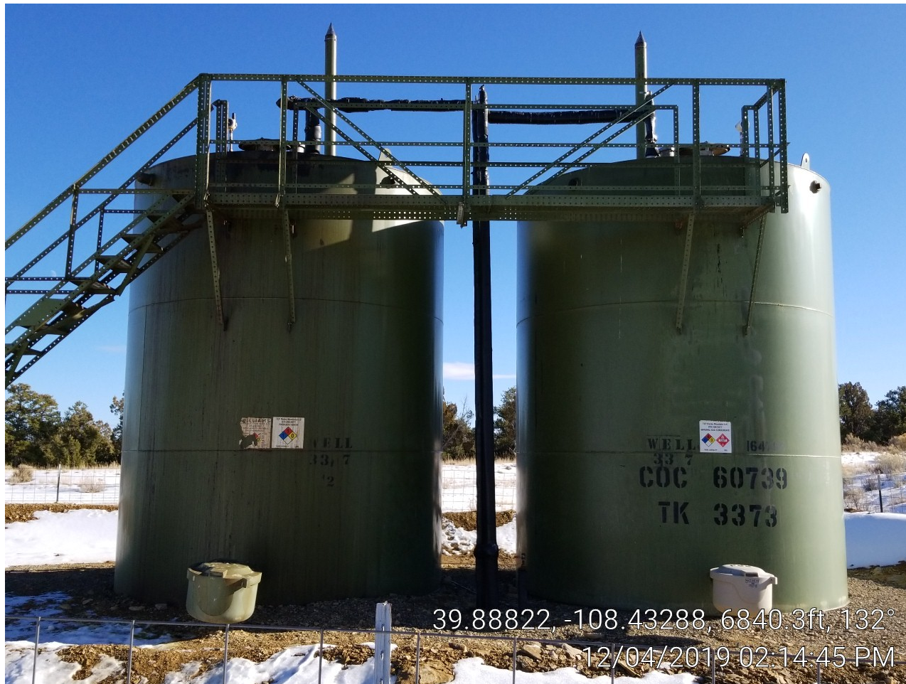
Photo 4. Tank battery.
