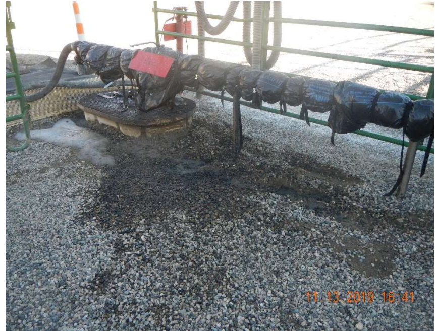
Photo #18 - View of the impacted soil around the load out area.
