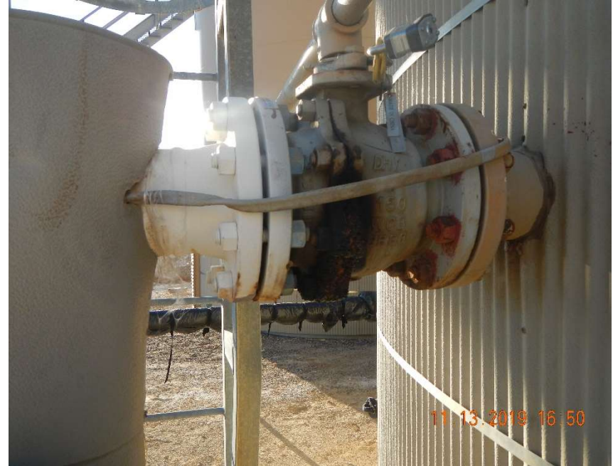
Photo #22 – View of the valve covered in a layer of hydrocarbons.
