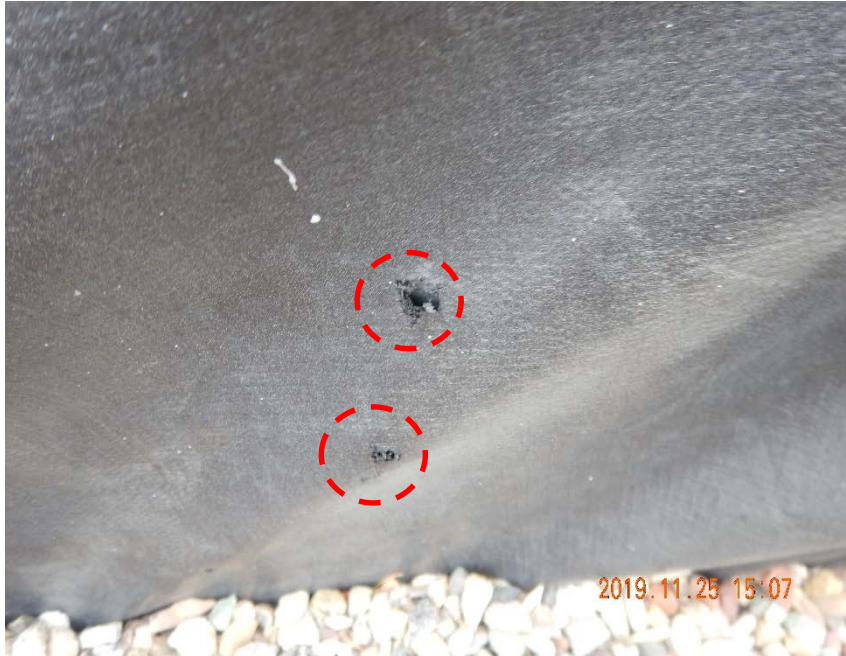
Photo #19 – Pinholes (red circles) observed in tank battery liner along south wall (4).
