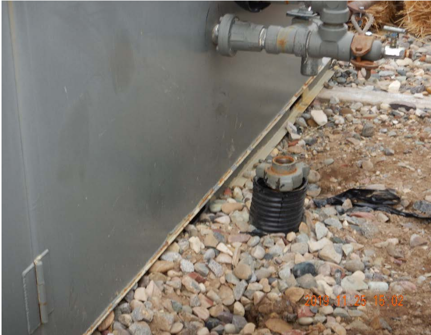
Photo #7 - Uncapped, unused 2" flowline risers located on north sides of separators (3).
