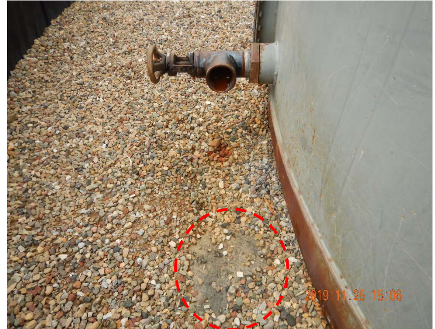
Photo #14 – View of valve on south side of tank. Note section of visible liner (red circle).
