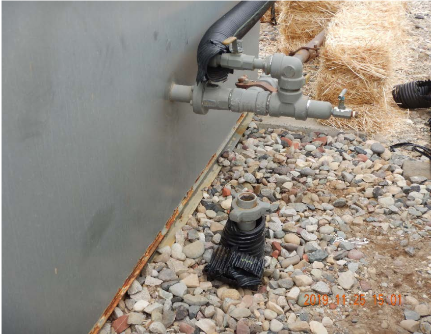
Photo #5 – Uncapped, unused 2” flowline risers located on north sides of separators (1).
