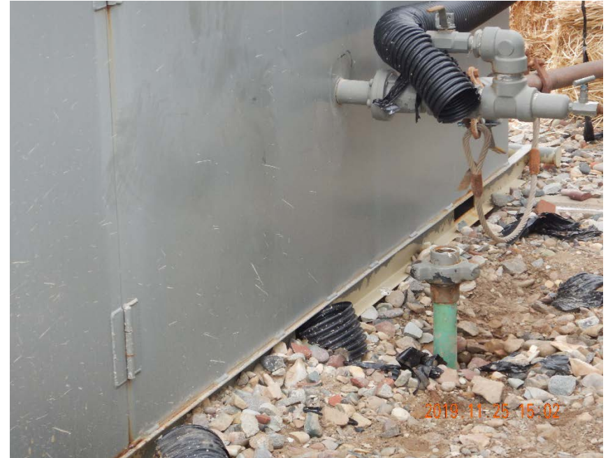
Photo #6 - Uncapped, unused 2” flowline risers located on north sides of separators (2).
