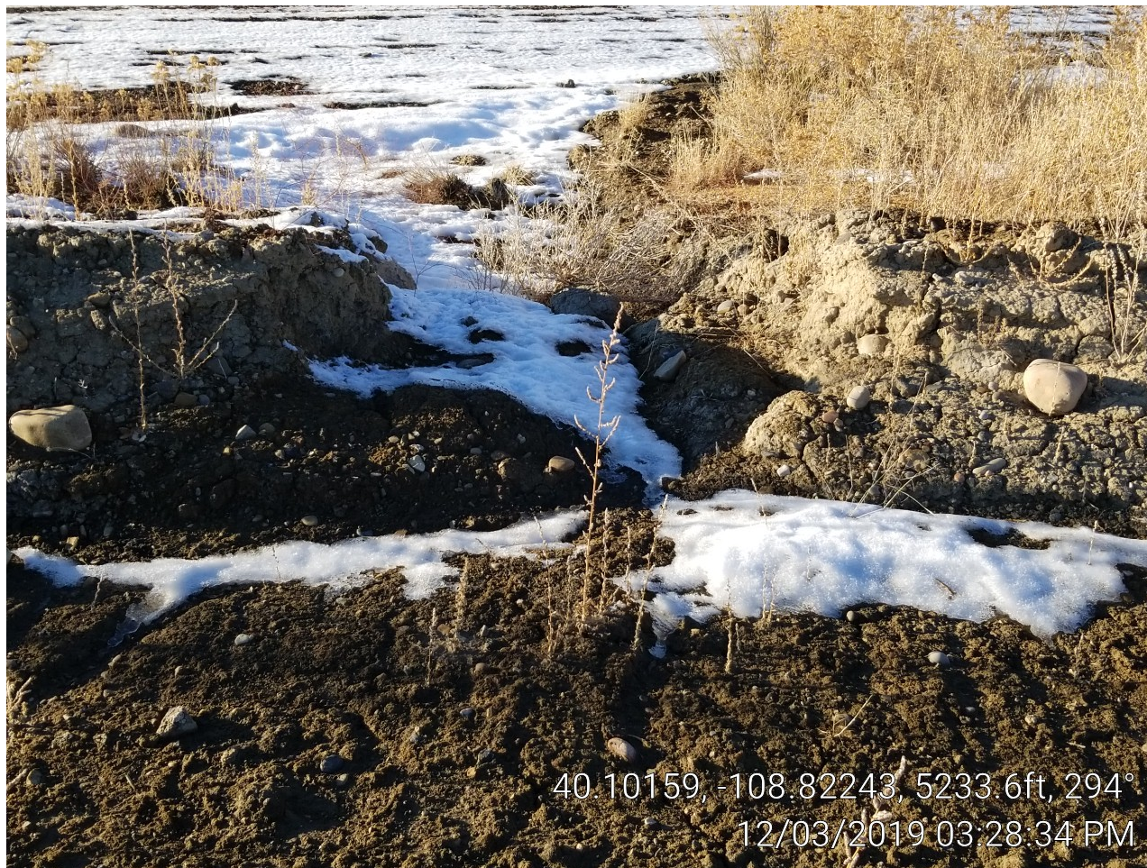
Photo 2. Break in location berm.
