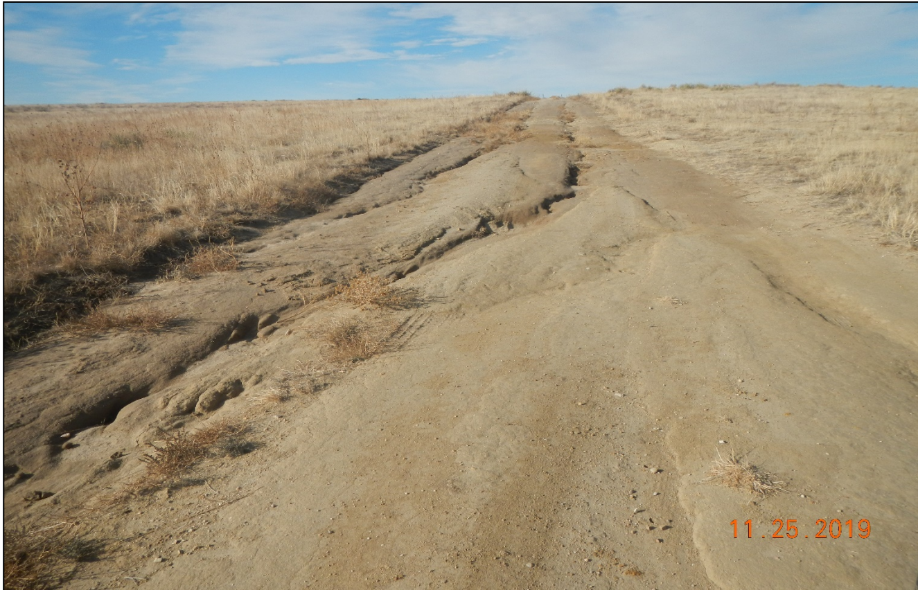
Photo 1. Facing west along the access road toward the location. There is erosion occurring down the road which is not maintained.
