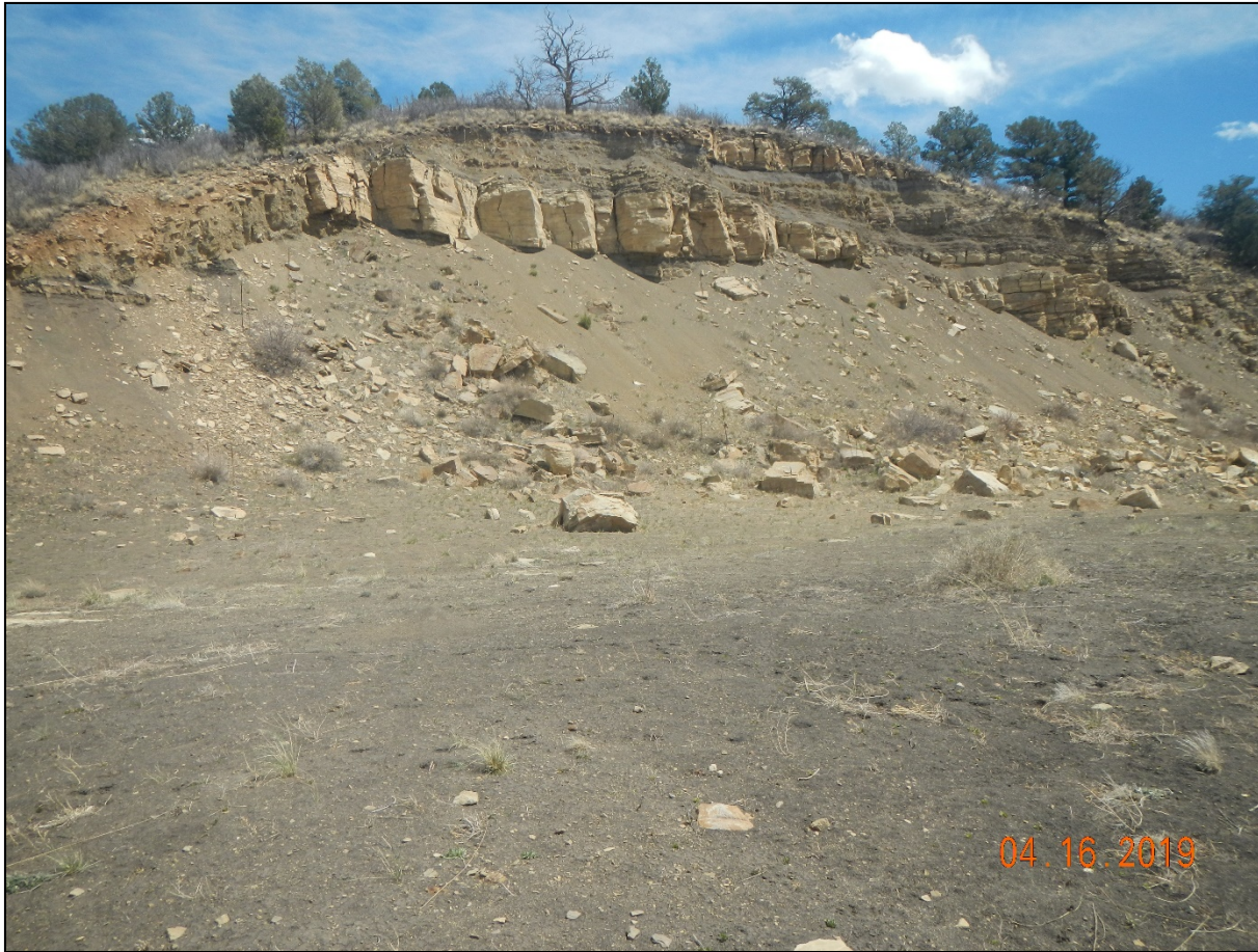
Photo 7. Facing towards the unstable vertical cut slope. Estimated to be 75' high.
