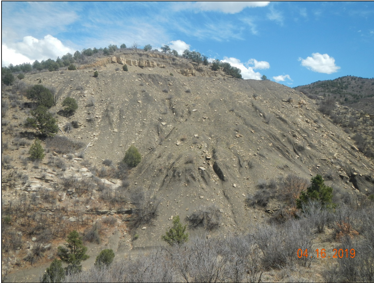
Photo 13. Facing east toward the location from across the canyon. The fill slope is not stabilized and shows signs of erosion. Location not recontoured.
