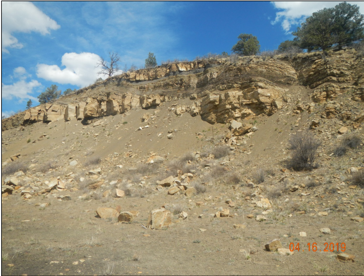
Photo 12. Facing towards the unstable vertical cut slope. Estimated to be 75' high.
