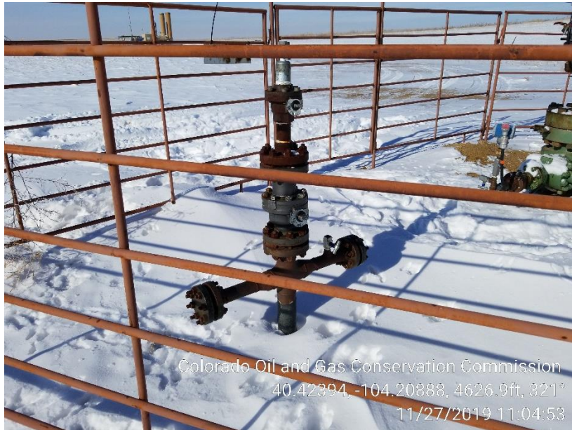
Photo 3 – Unmarked 3" Riser at Wellhead
