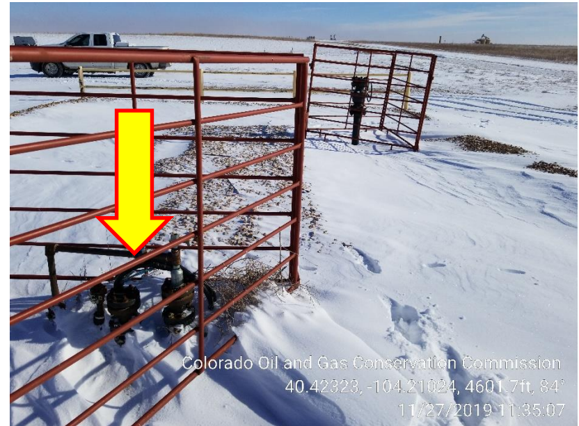
Photo 4 – Unmarked Riser on South side of location
