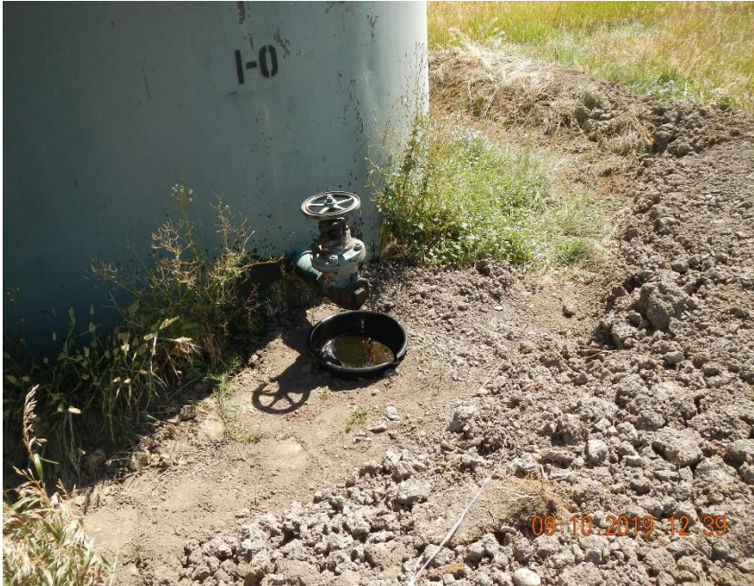
Recently constructed secondary containment berm around AST. Drip pan beneath load out valve.
