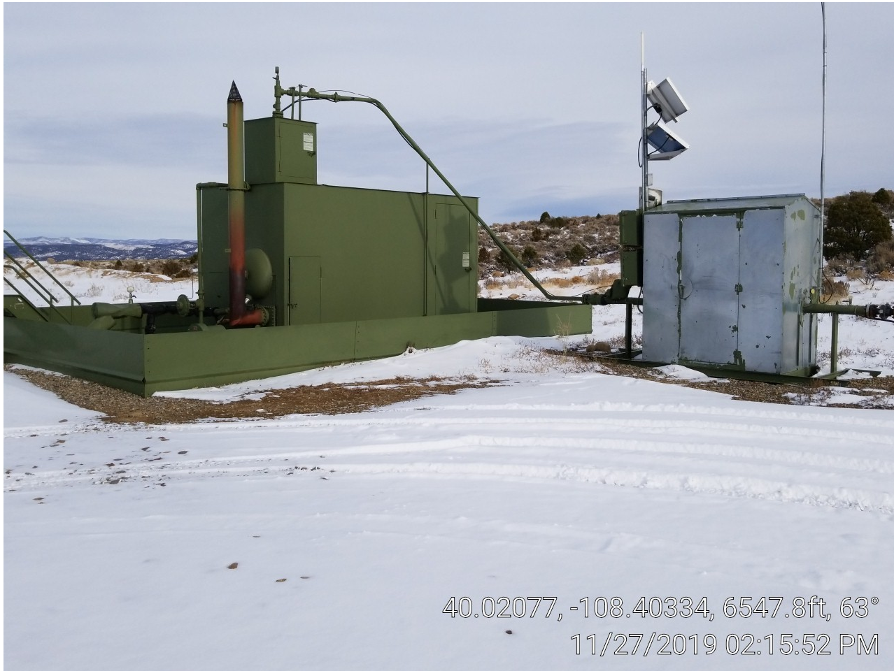
Photo 2. Separator & gas meter building.
