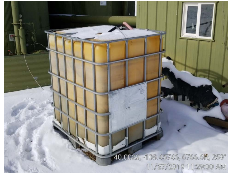
Photo 5. Container with no secondary containment.
