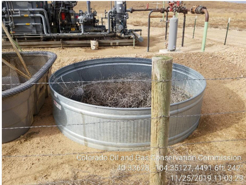
Photo 3 – Debris inside Secondary Containment and Wildlife Netting is in disrepair.
