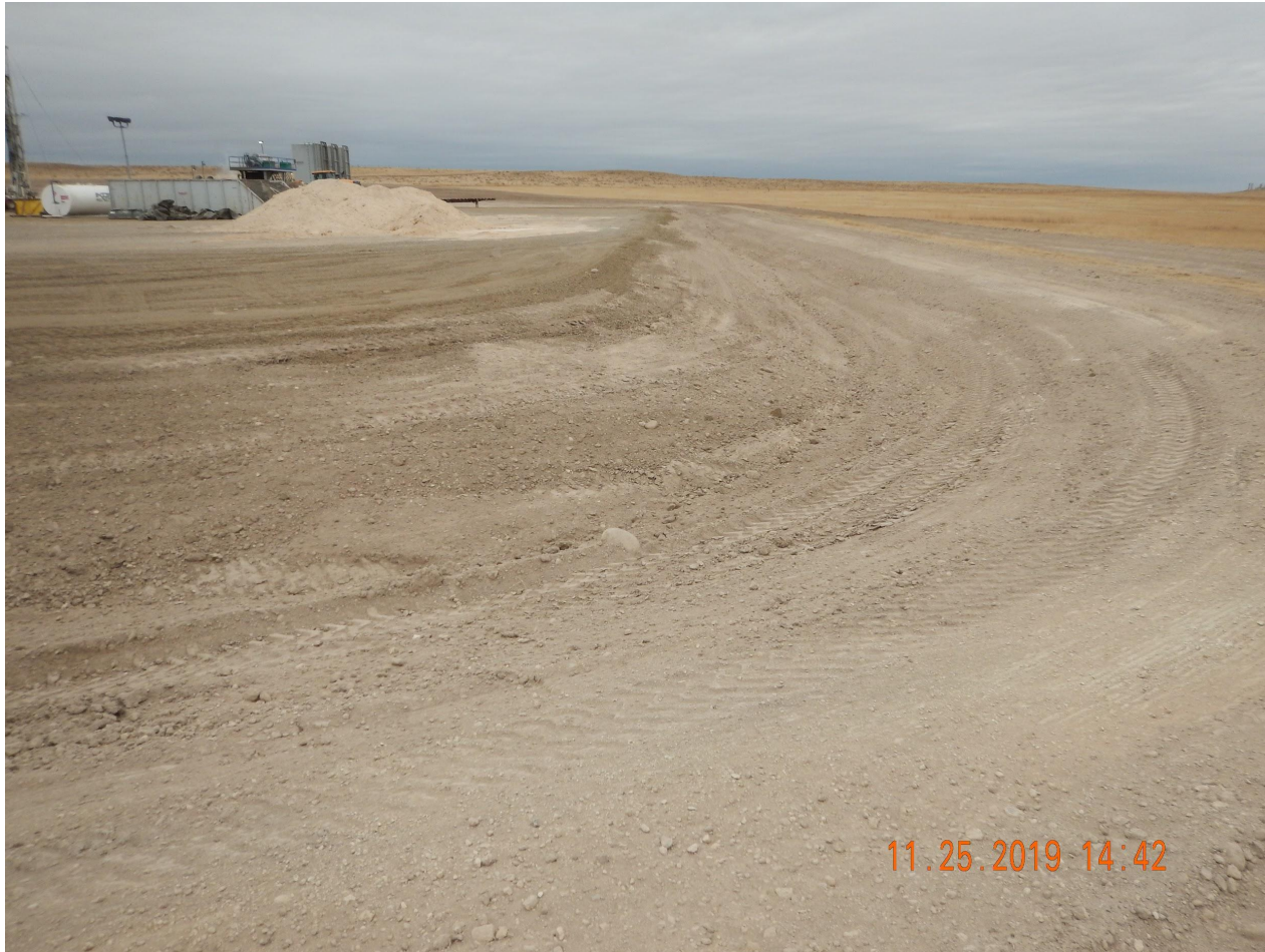
Photo 5. Photo taken from the northeastern perimeter of location, facing West. Photo illustrates the ditch BMP around the entire well pad perimeter.
