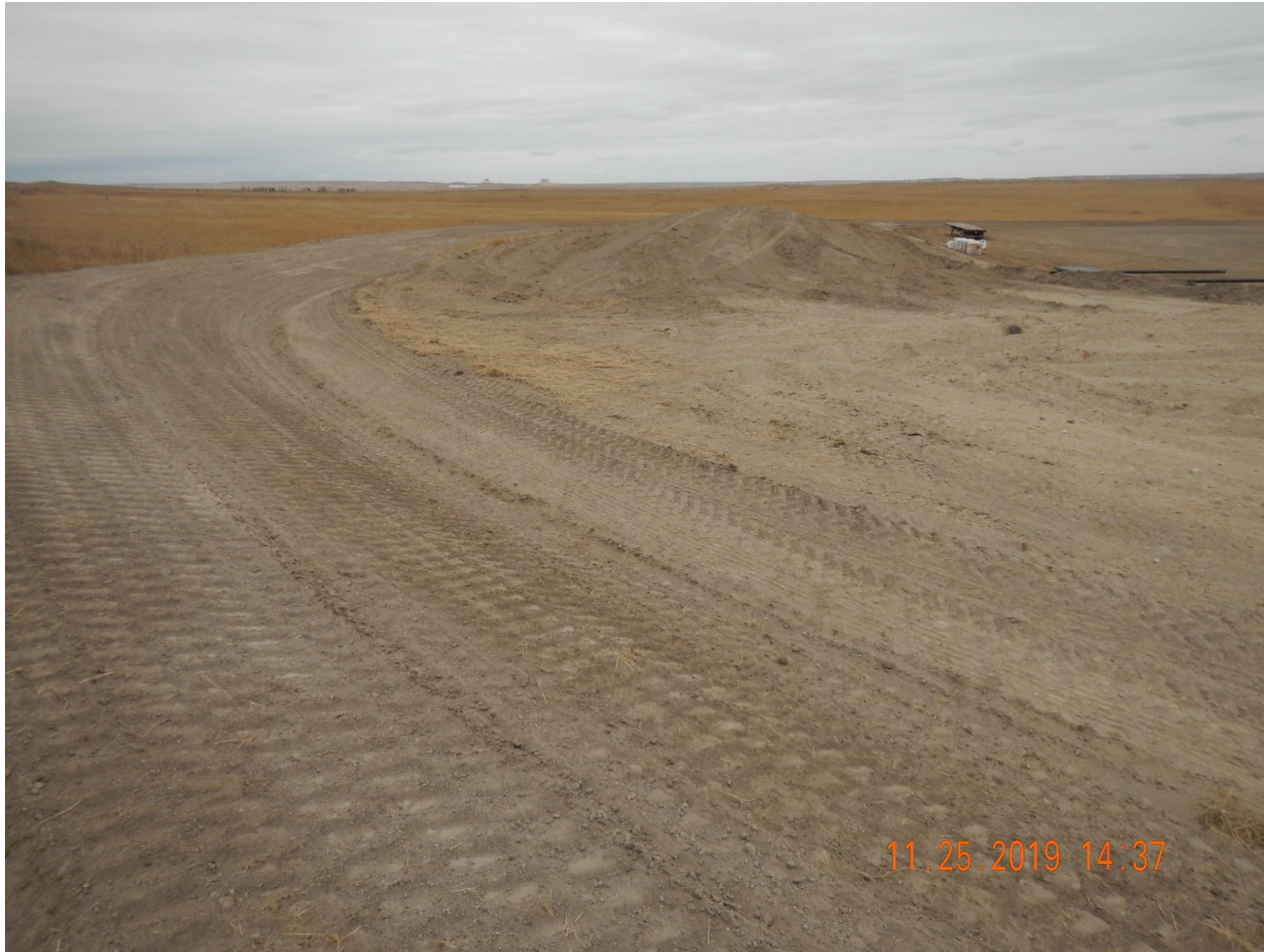
Photo 2. Photo taken from the southwestern perimeter of location, facing North. Photo illustrates a ditch and berm BMP installed around the entire perimeter of location. Also, photo illustrates the second soil stockpile that has been temporarily stabilized with equipment tracking.
