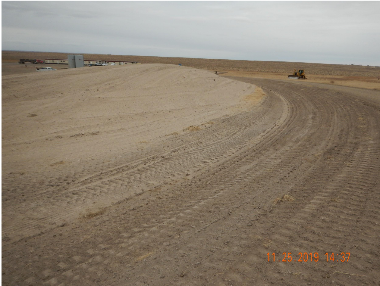
Photo 1. Photo taken from the southwestern perimeter of location, facing East. Photo illustrates a ditch and berm BMP installed around the entire perimeter of location. Operator also has another ditch BMP along portions of the western, northern and eastern well pad. Also, photo illustrates one of two soil stockpiles that have been temporarily stabilized with equipment tracking.
