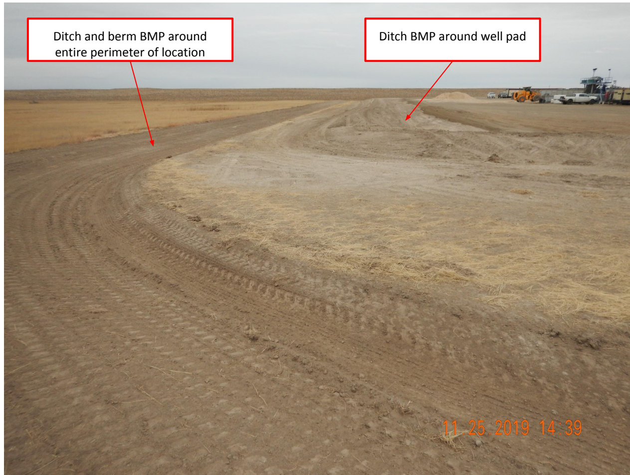
Photo 4. Photo taken from the northwestern perimeter of location, facing East. Photo illustrates a ditch and berm BMP installed around the entire perimeter of location.
