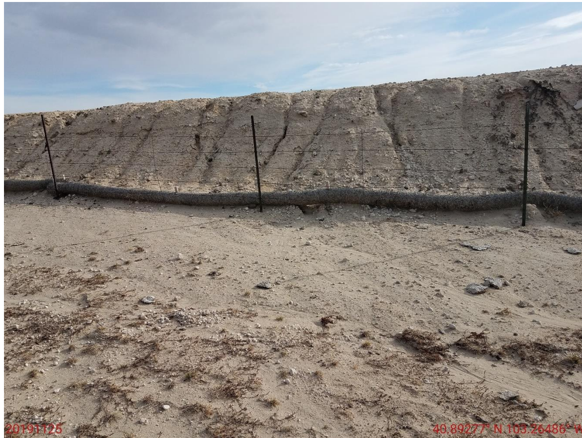
Photo 13: Photo taken from the southwest end of the pit, facing east. Photo shows erosion degradation and wattles in improper functioning condition.
