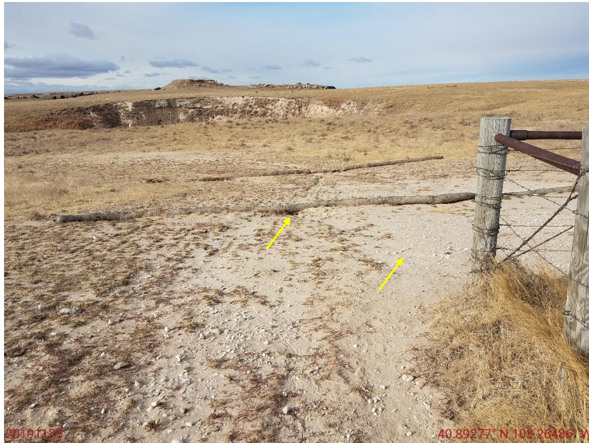
Photo 9: Photo taken from the southwest end of the pit, facing west. Photo shows areas where desirable vegetative establishment is not occurring, and erosion degradation.
