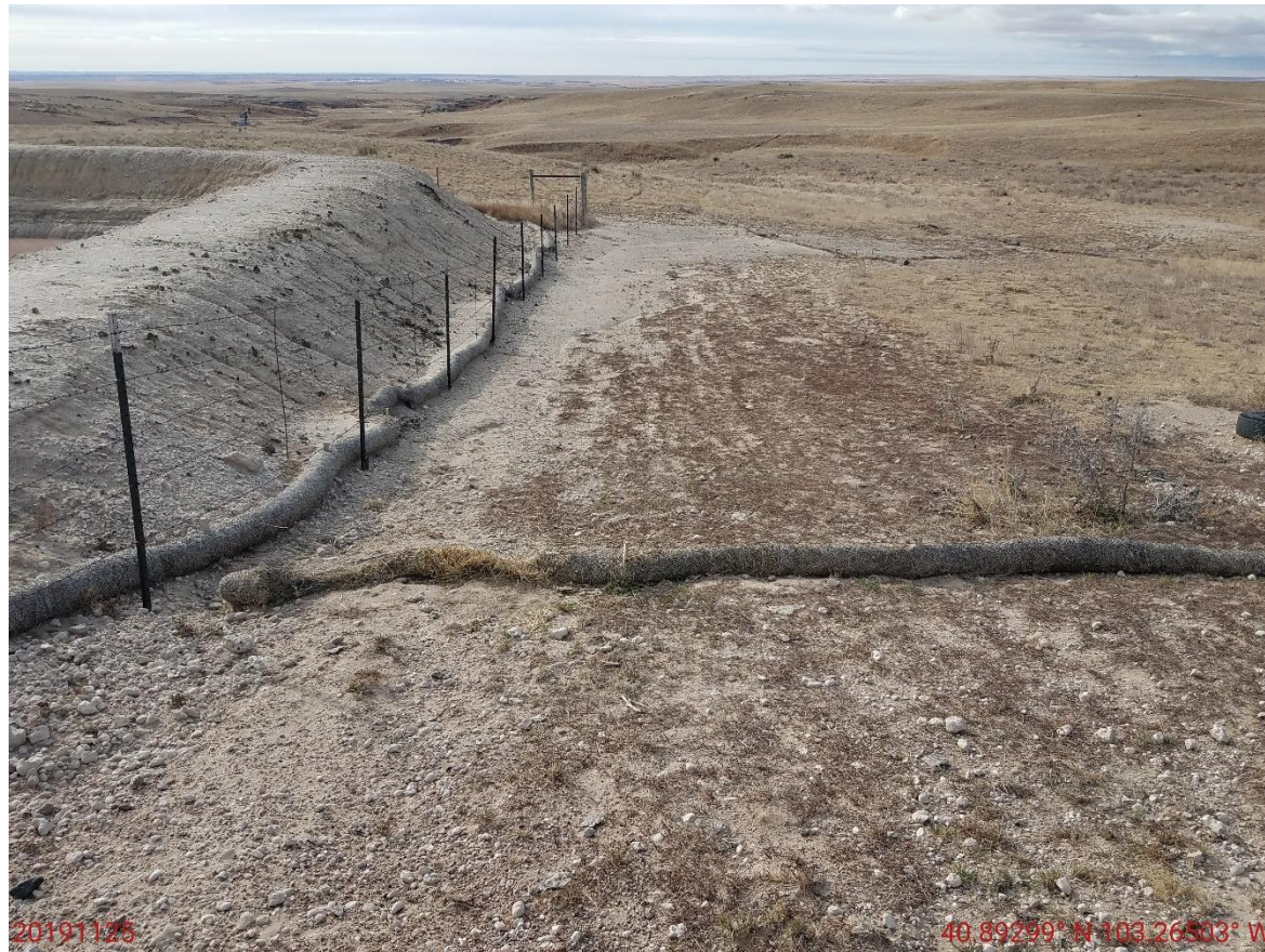
Photo 14: Photo taken from the southwest end of the location, facing south. Photo shows areas where desirable vegetative establishment is not occurring, and erosion degradation.
