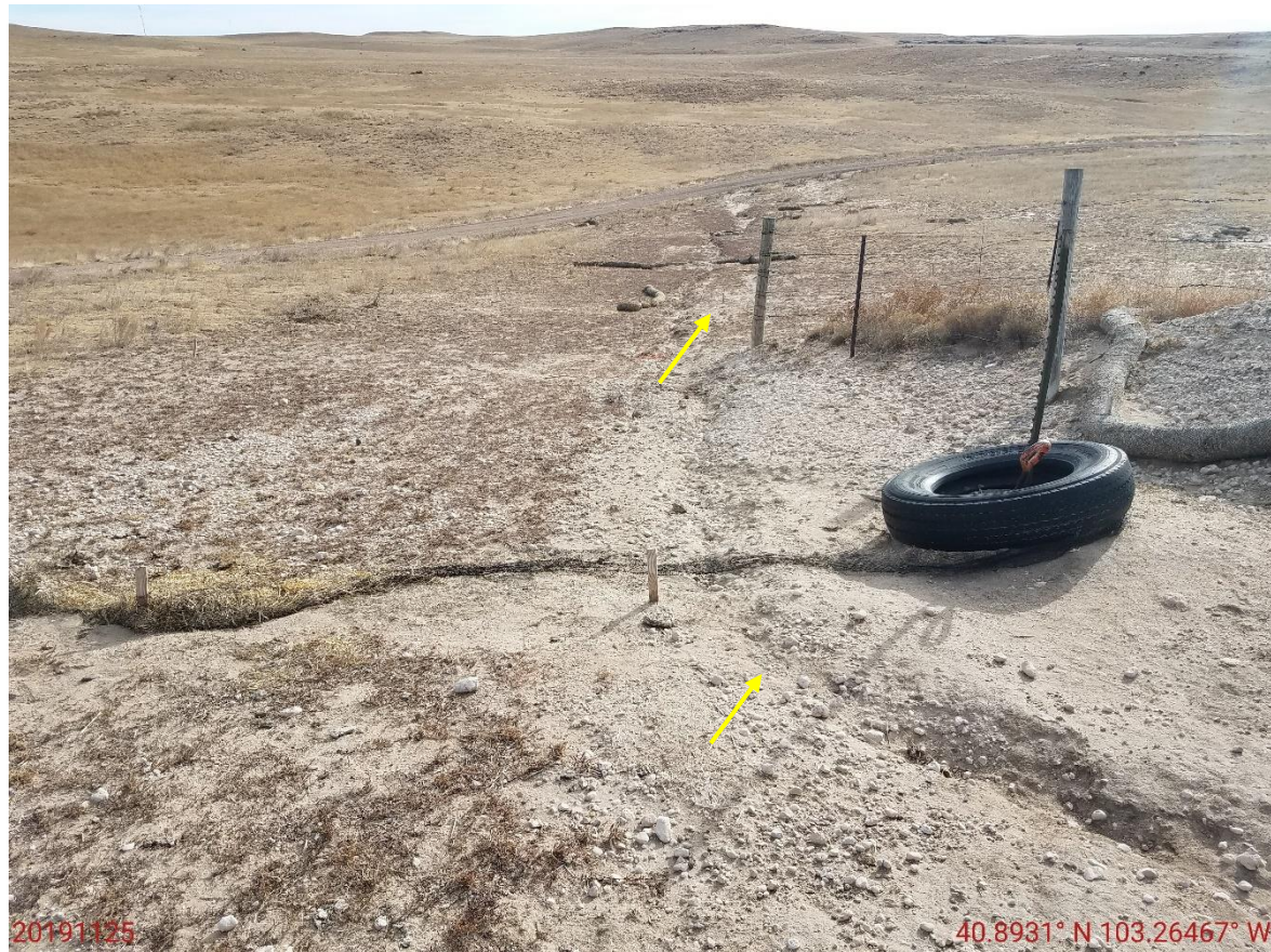
Photo 2: Continued from photo 1. Photo facing east. Photo shows stormwater erosion degradation has been allowed to continue on the location. Photo also shows wattles in disrepair and that no additional BMPs to stabilize the soils have been installed per corrective actions and 1002.f.
