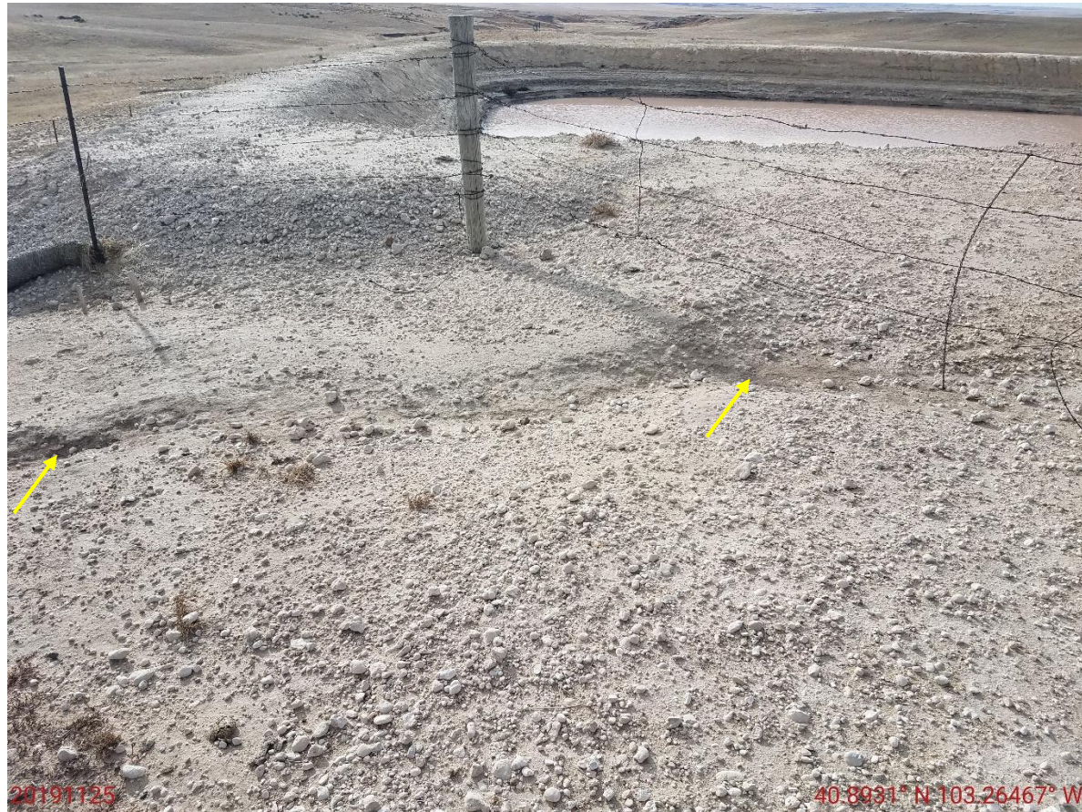
Photo 1: Photo taken from the east end of the location, facing south. Photo shows stormwater erosion degradation has been allowed to continue on the location.
