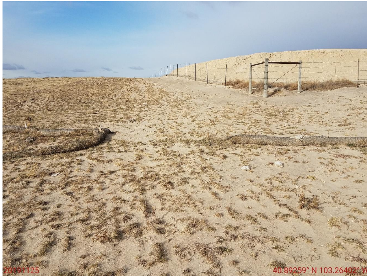
Photo 7: Photo taken from the southeast end of the pit, facing west. Photo shows straw wattles in disrepair; Operator failed to install BMP in accordance with good engineering practices.
