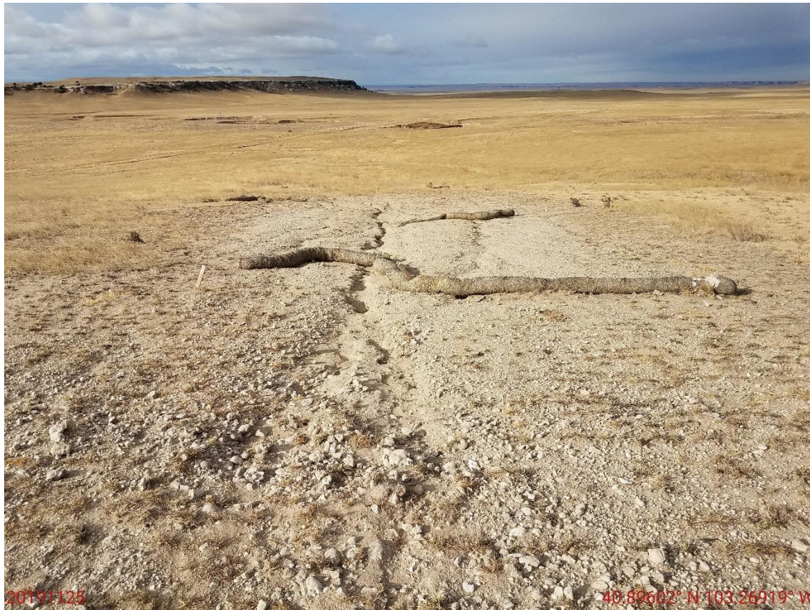
Photo 15: Photo taken from the west of the pit, facing west. Photo shows erosion degradation and wattle debris.
