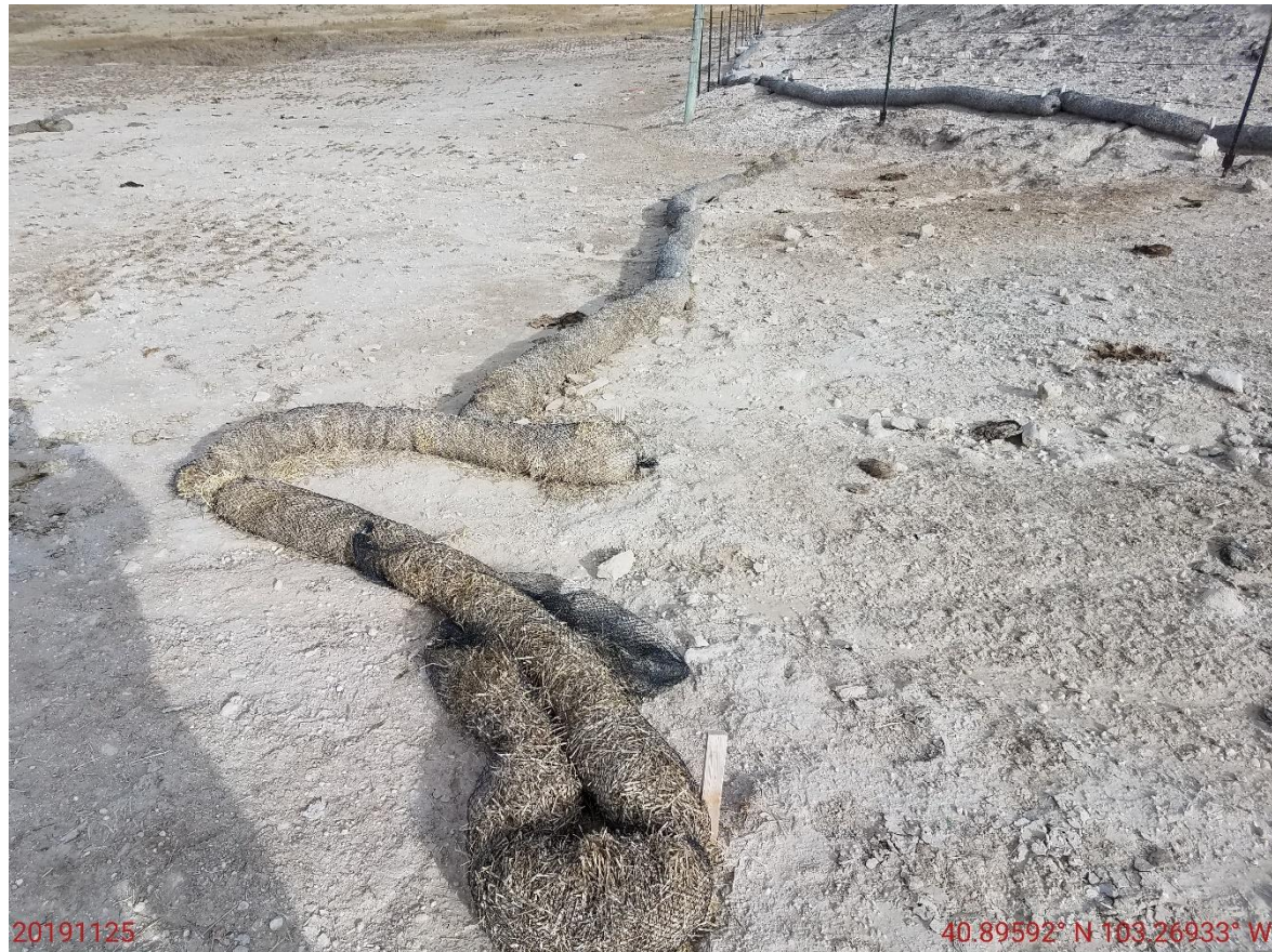
Photo 13: Photo shows wattle in disrepair. This is considered debris.
