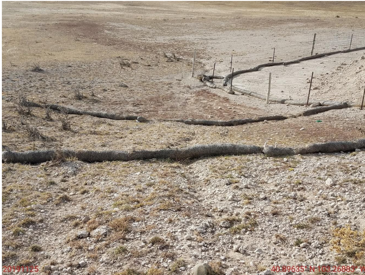
Photo 4: Photo taken from the south end of the production area, facing southwest. Previous inspections documented that wattle BMPs have not been installed in accordance with good engineering practices, and that no stabilization BMPs have been installed per CAs. Photo shows BMPs remain insufficient and erosion degradation has been allowed to continued.
