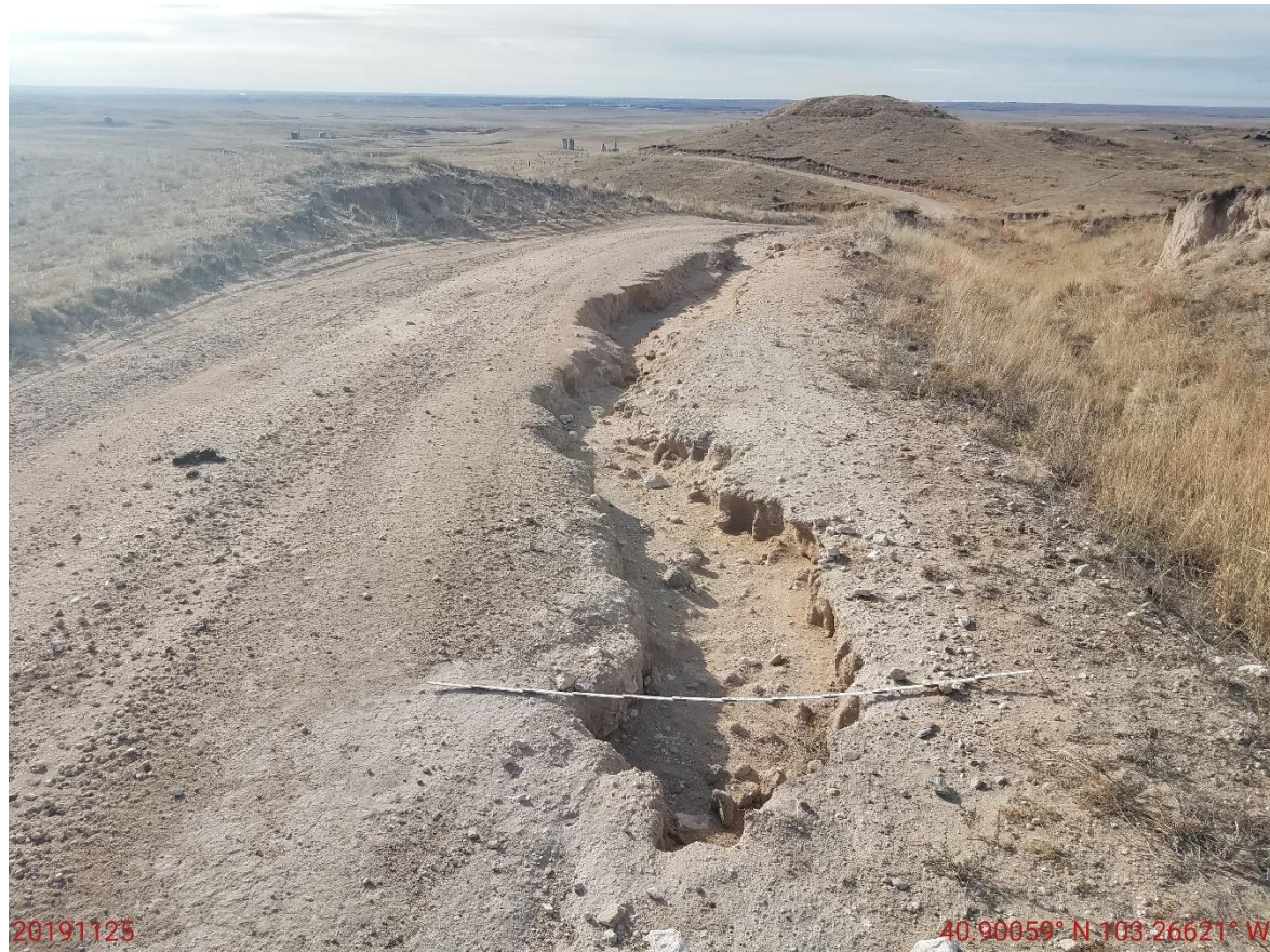
Photo 22: Photo taken from the access road north of the location, facing south. Photo shows erosion degradation on the access road. 6 foot measuring stick for reference.
