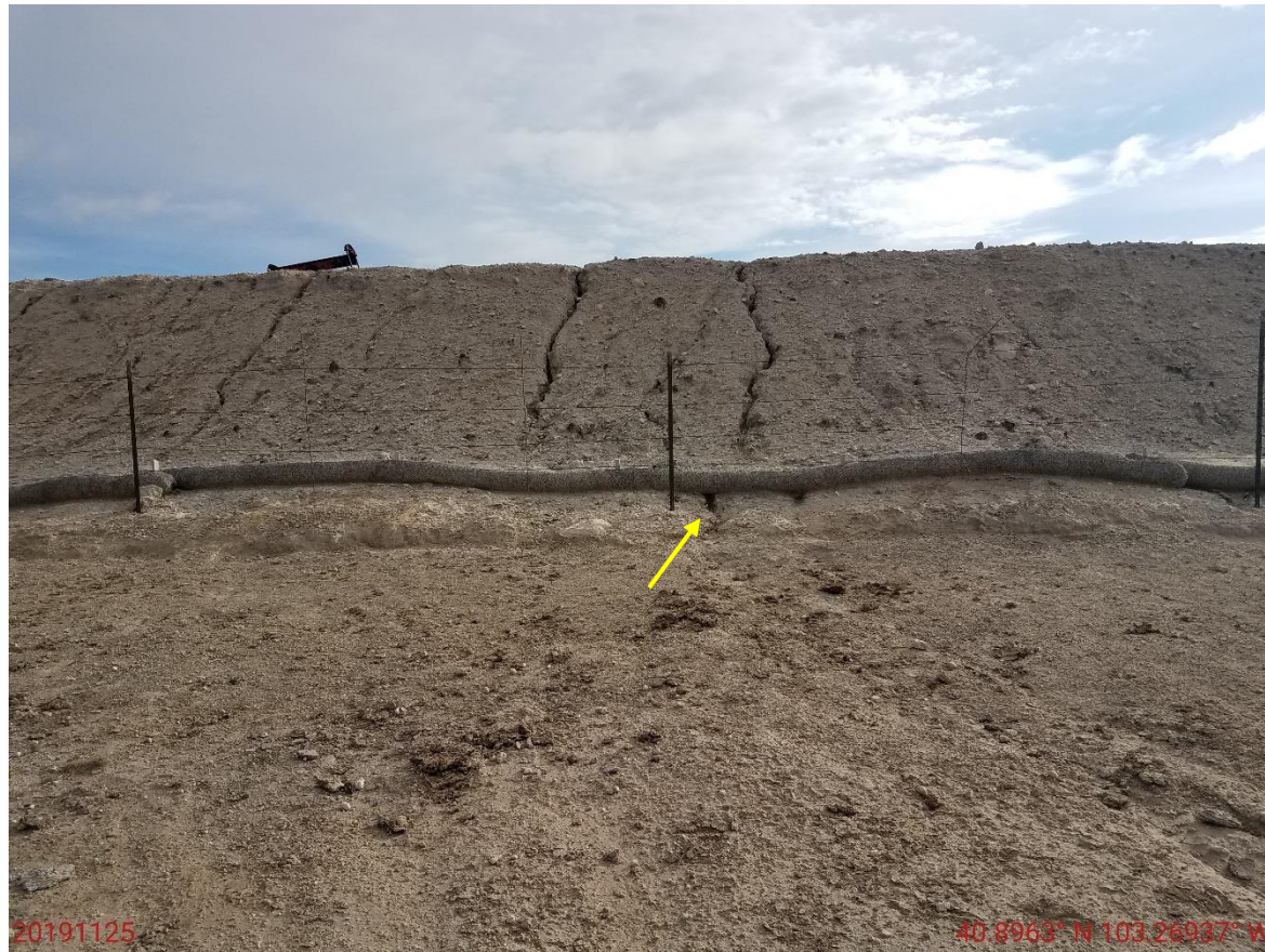
Photo 19: Photo taken from the west end of the pit, facing east. Photo shows erosion degradation from the pit. Photo also shows wattles were not installed in accordance with good engineering practices, resulting in failure of the BMP.
