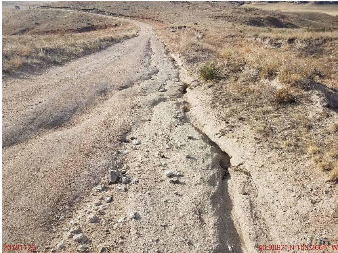
Photo 23: Photo taken from the access road north of the location, facing south. Photo shows erosion degradation on the access road. 6 foot measuring stick for reference.
