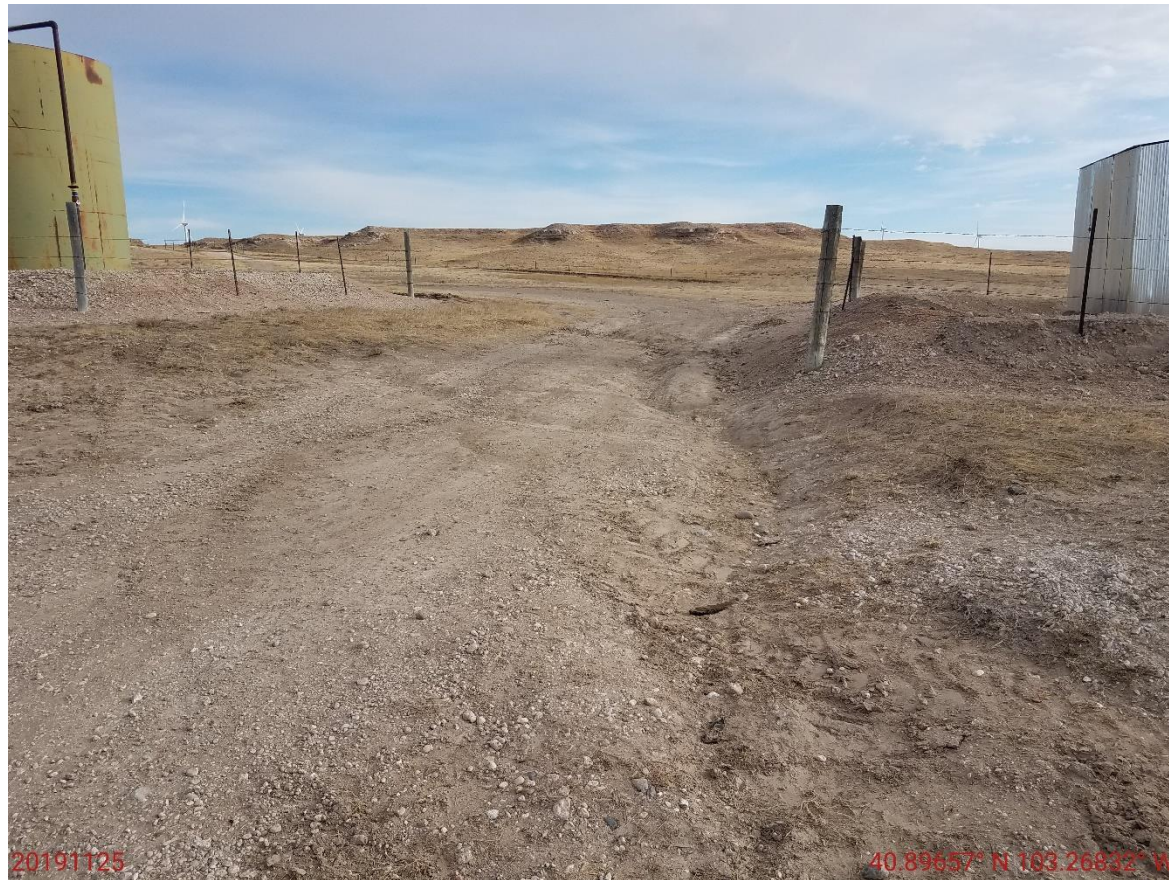
Photo 21: Photo taken from the southeastern area of the pad. Photo shows erosion degradation on access road.
