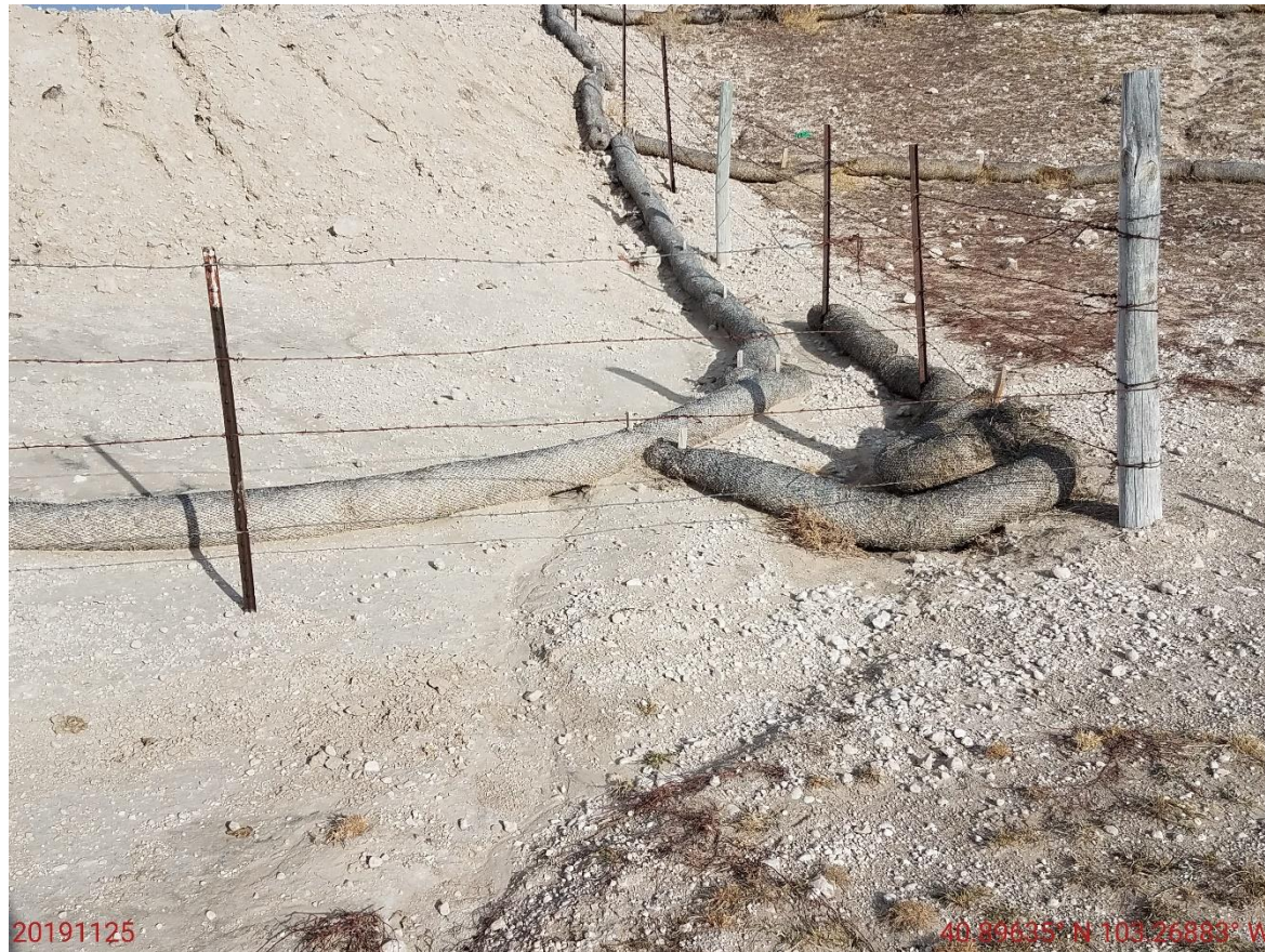
Photo 8: Photo taken from the south end of the pit. Photo shows straw wattles around pit. Previous inspections documented that wattle BMPs were not installed in accordance with good engineering practices. Photo shows wattles remain improperly installed. Many wattles have been “blown out” and are now debris.
