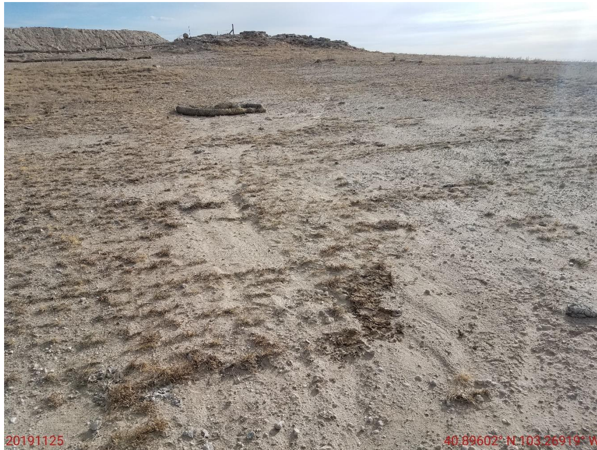
Photo 14: Photo taken from the west of the pit, facing east. Photo shows wattles have not been maintained, and stormwater erosion degradation has been allowed to continue.
