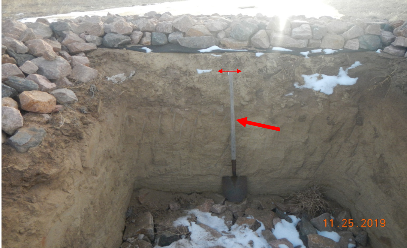
Photo 4. The sediment trap was not installed in accordance to good engineering practice. The arrow points to a 4'8" shovel placed in the sediment trap. The 3 sides of the sediment trap are vertical and per good engineering practice, should not be installed steeper than 2:1 slope.
