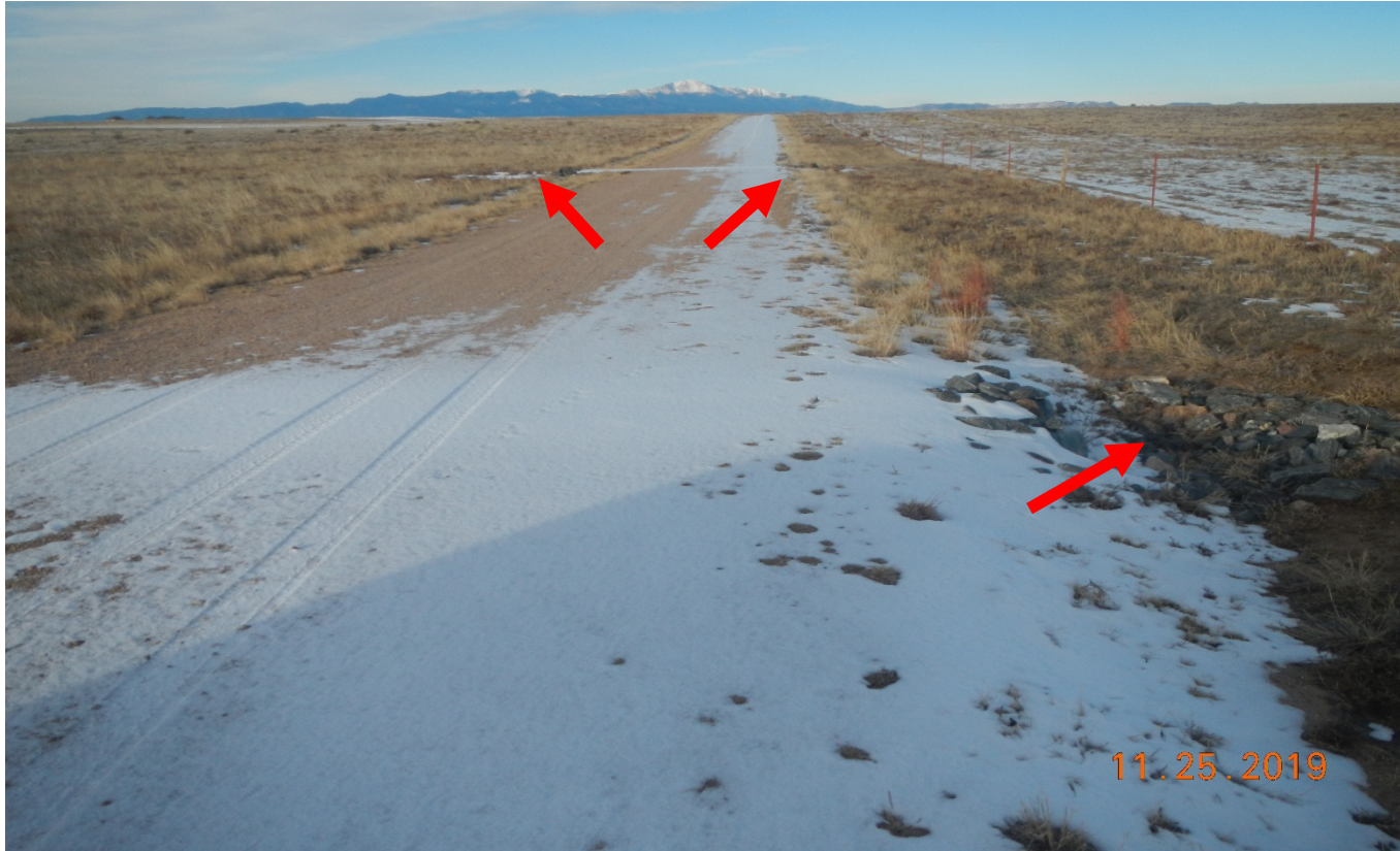
Photo 9. Facing west along the access road . There are culverts at this area of the road with inlet and outlet protection installed shown by red arrows. This photo depicts compliance of the corrective action.
