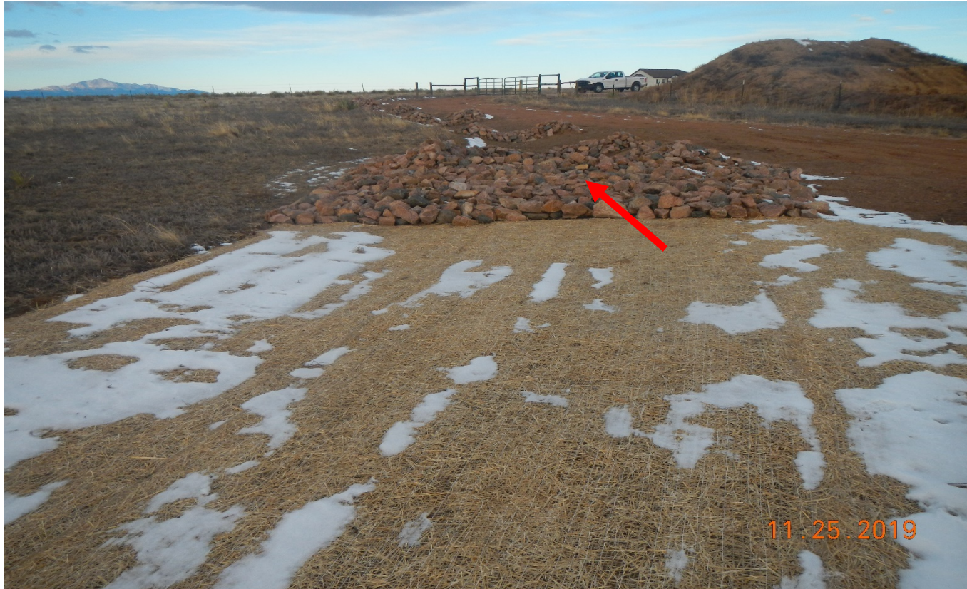
Photo 6. Facing northwest toward the road. Sediment trap is located where red arrow is shown. Rock check dams are installed further up along the road toward the gate.
