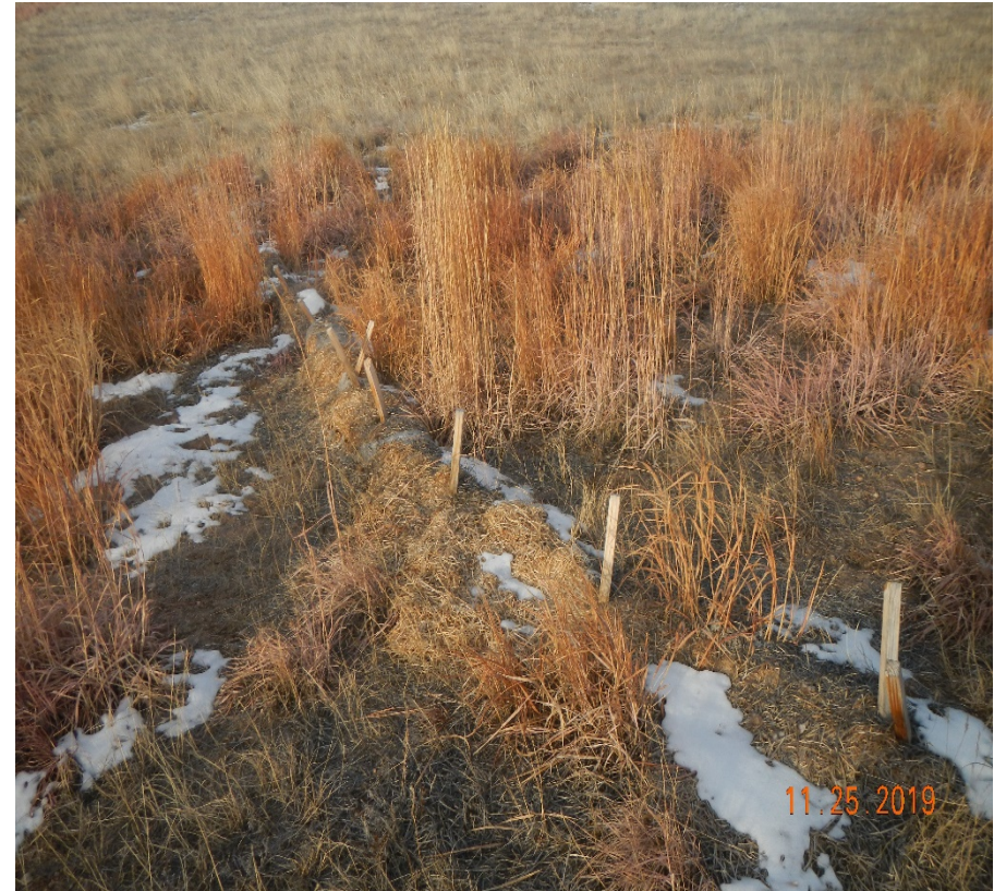
Photo 12. Wattles installed at the location have degraded and need to be removed or replaced. The left photo shows the wattles in the previous inspection on 7/25/2019. The right photo taken 11/25/2019 shows the same degraded wattles remain. The photos depict noncompliance of the corrective action.
