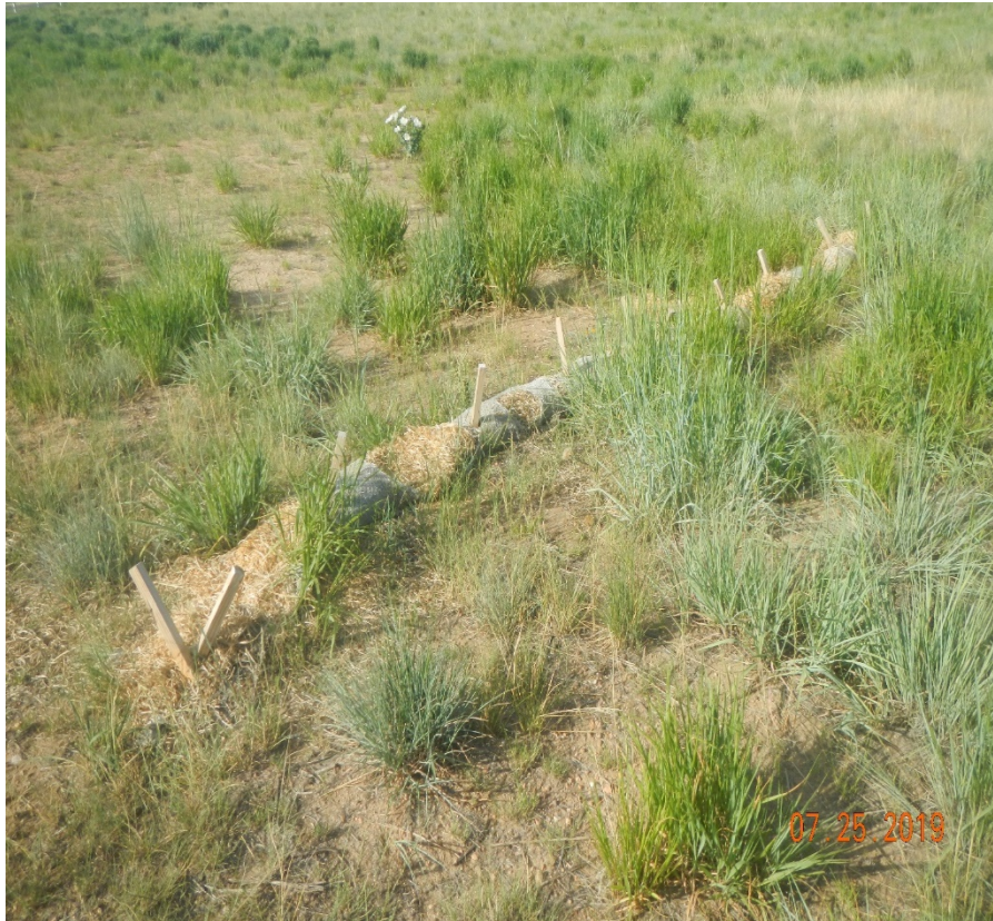
Photo 12. Wattles installed at the location have degraded and need to be removed or replaced. The left photo shows the wattles in the previous inspection on 7/25/2019. The right photo taken 11/25/2019 shows the same degraded wattles remain. The photos depict noncompliance of the corrective action.
