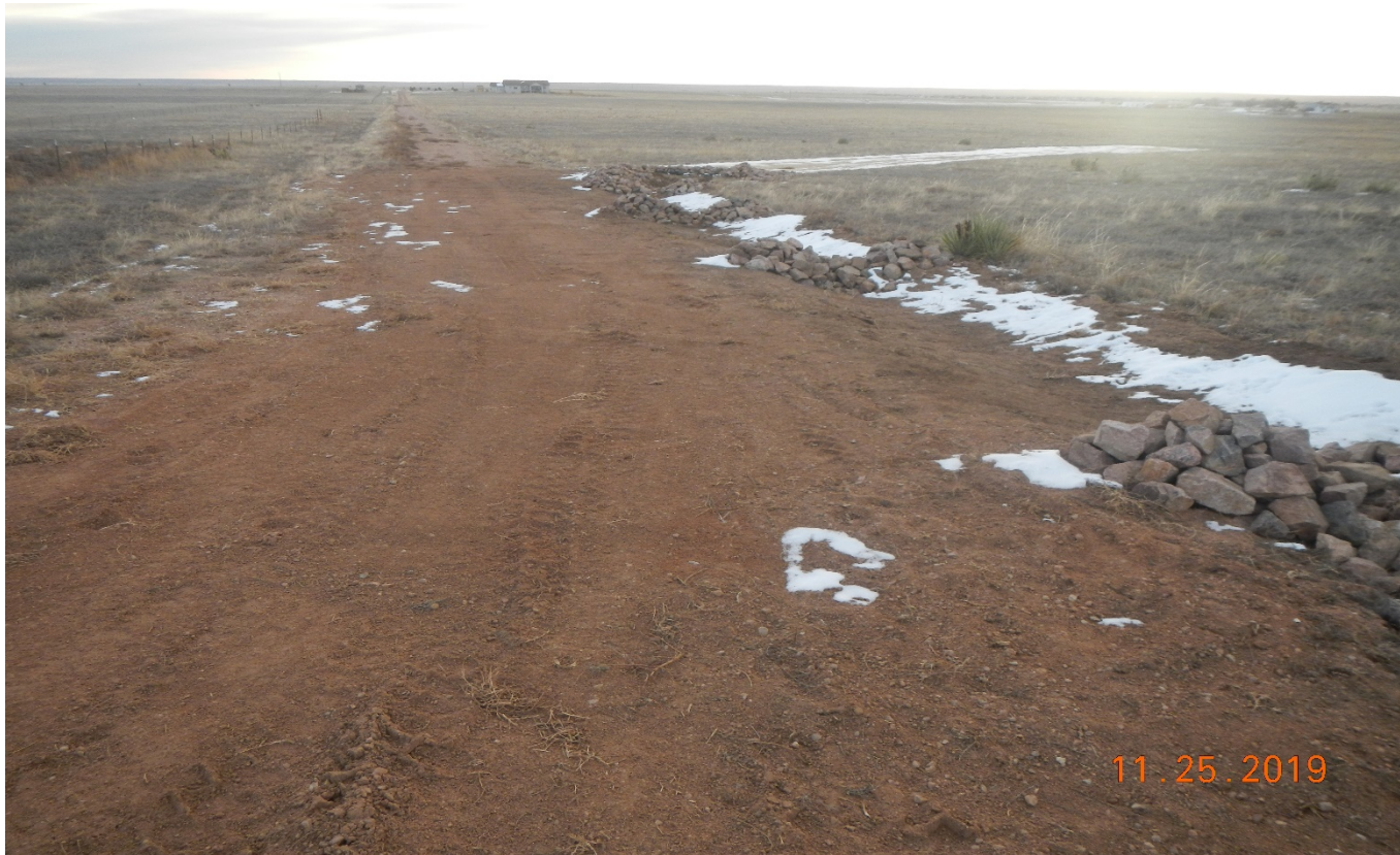
Photo 1. Facing east on the access road. Rock rip/rap check dams have been installed along the road since the previous inspection. The center of the check dams are at least 6 inches lower than the edges as required.
