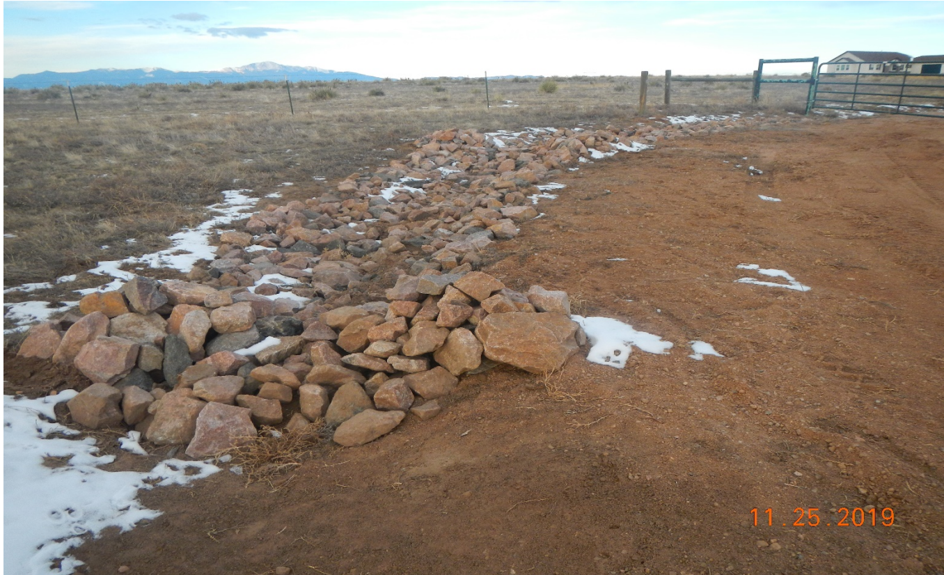
Photo 7. Rock rip/rap was installed along the road near the double gates. This photo depicts compliance of the corrective action.
