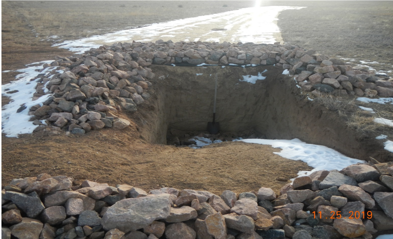
Photo 3. The sediment trap was not installed in accordance to good engineering practice. The depth of the spillway should be 1 ft. below the low point of the embankment.
