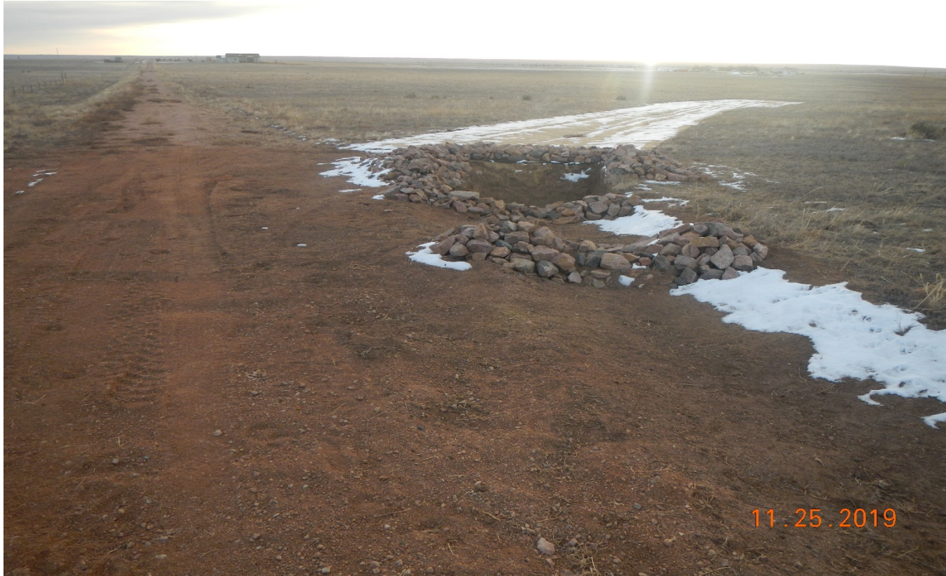
Photo 2. Facing southeast toward the area of erosion which extended out into the pasture which was identified in the previous inspections. The erosion in the pasture has been reclaimed. Rock check dams and a sediment trap have been installed since the previous inspection.
