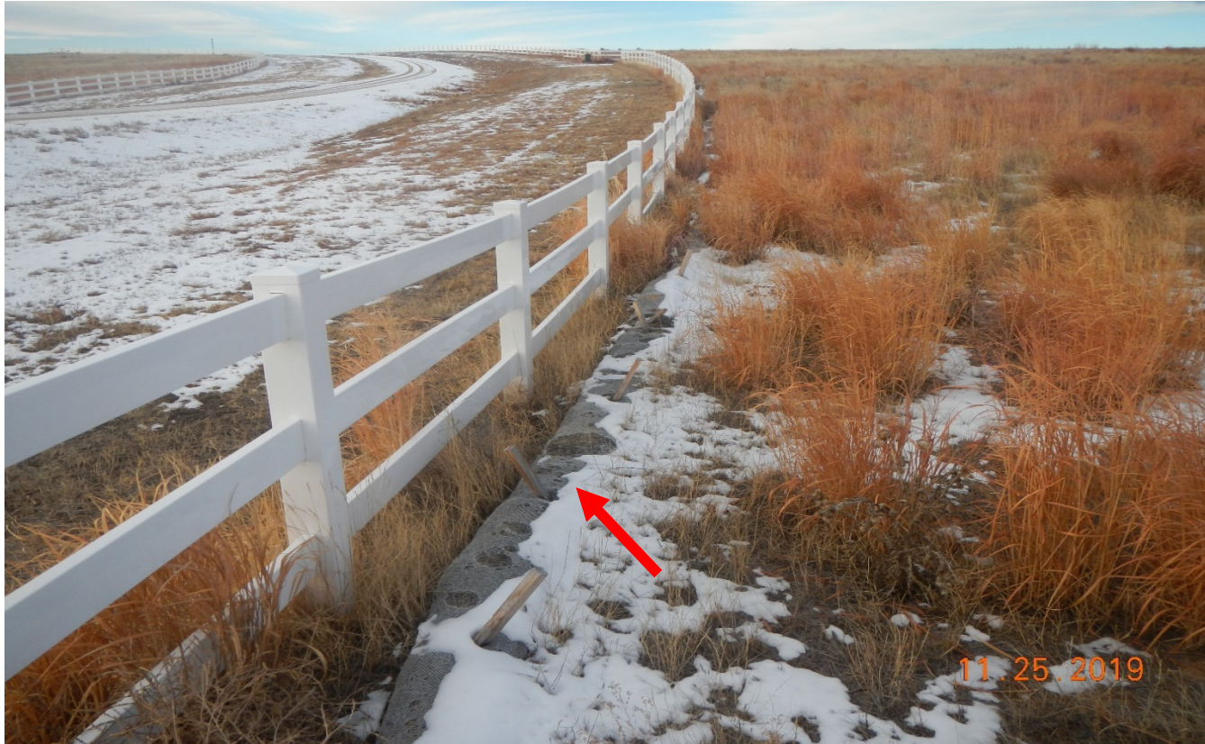
Photo 14. The degraded wattles have not been removed since the previous inspection. The photo depicts noncompliance of the corrective action.
