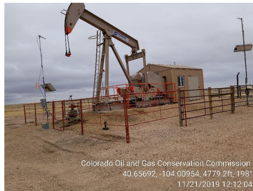
Photo 2 – Stained Soil at Wellhead, Unused Wellhead parts, Unmarked 2" Riser
