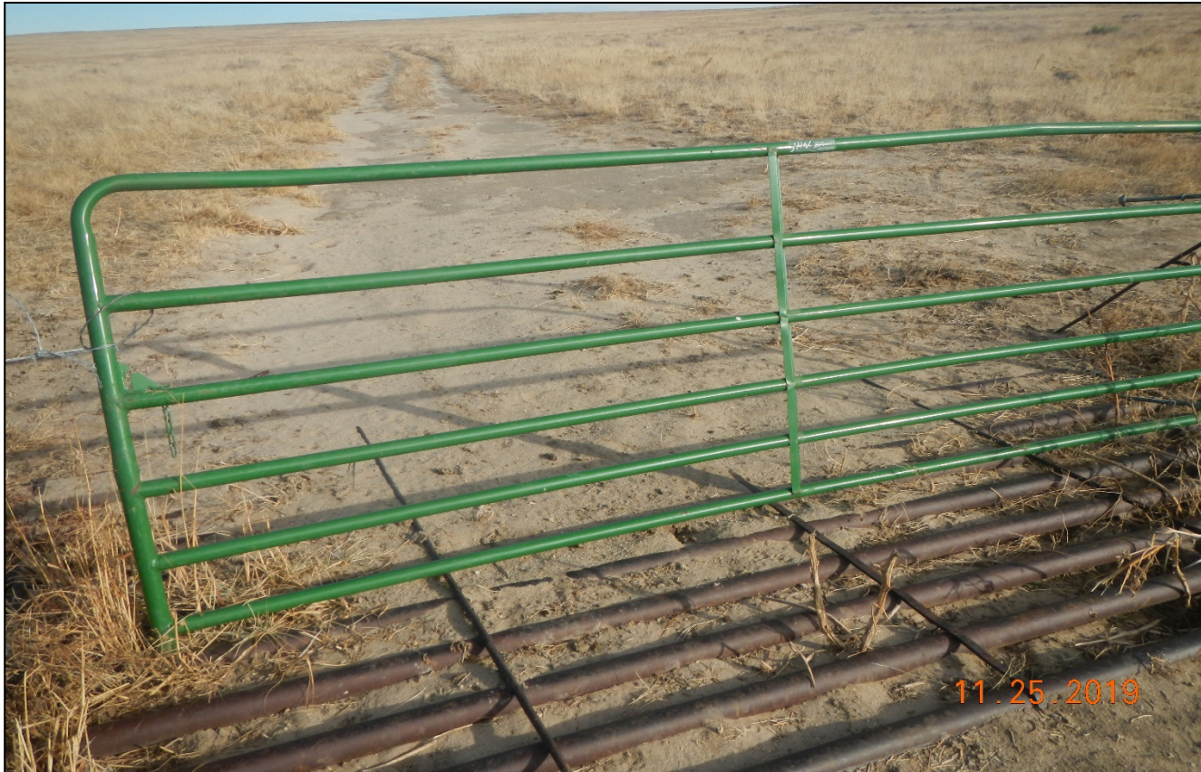
Photo 1. Facing north at the beginning of the access road. The cattle guard has filled in with sediment and needs maintenance.
