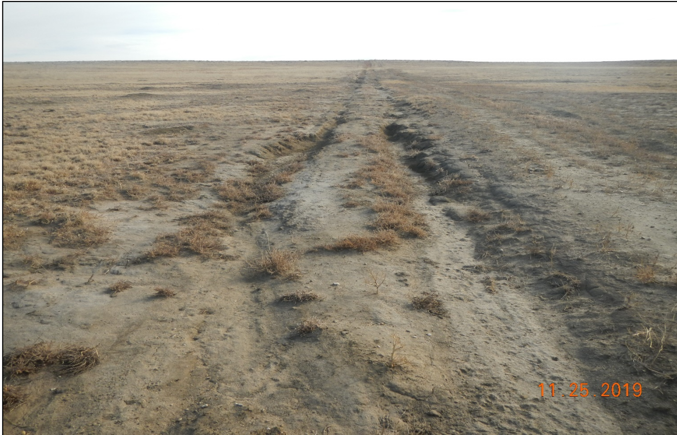
Photo 1. Facing east along the access road which was requested to remain. There are erosion issues along the road that need to be repaired and stabilized. Previous corrective action was not performed.
