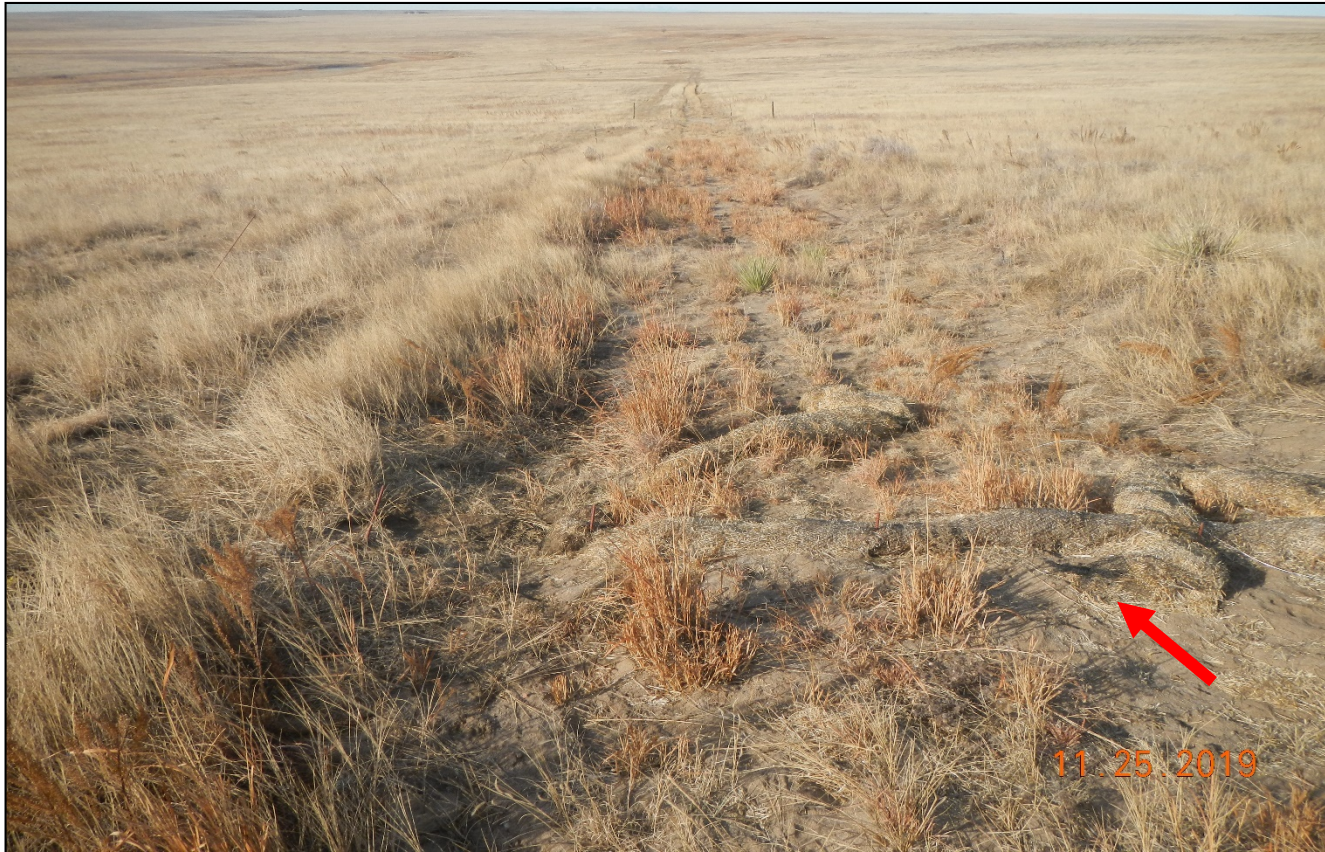
Photo 5. Facing back to the west at the reclaimed portion of the access road. Arrow points to wattles that are not maintained. The photo depicts noncompliance of the corrective action.
