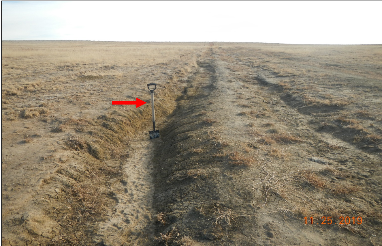
Photo 2. Facing east along the access road which was requested to remain. There are erosion issues along the road that need to be repaired and stabilized. Arrow points to 3.5 ft. shovel to show depth of erosion. Previous corrective action was not performed.
