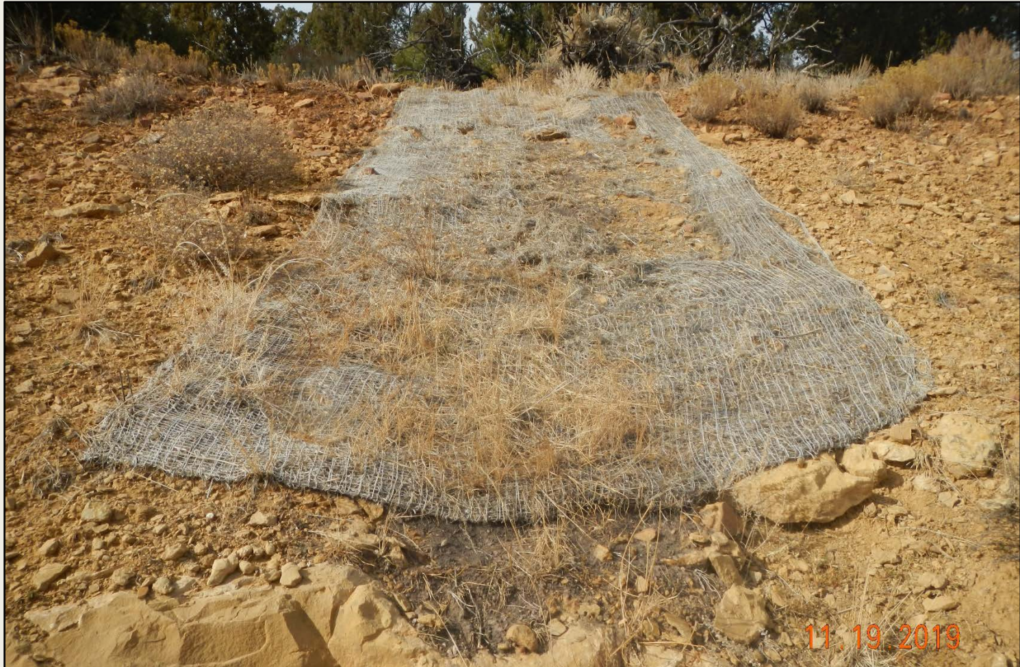
Photo 5. View of another erosion blanket on the cut-slope. A portion of the blanket is torn and needs repair.
