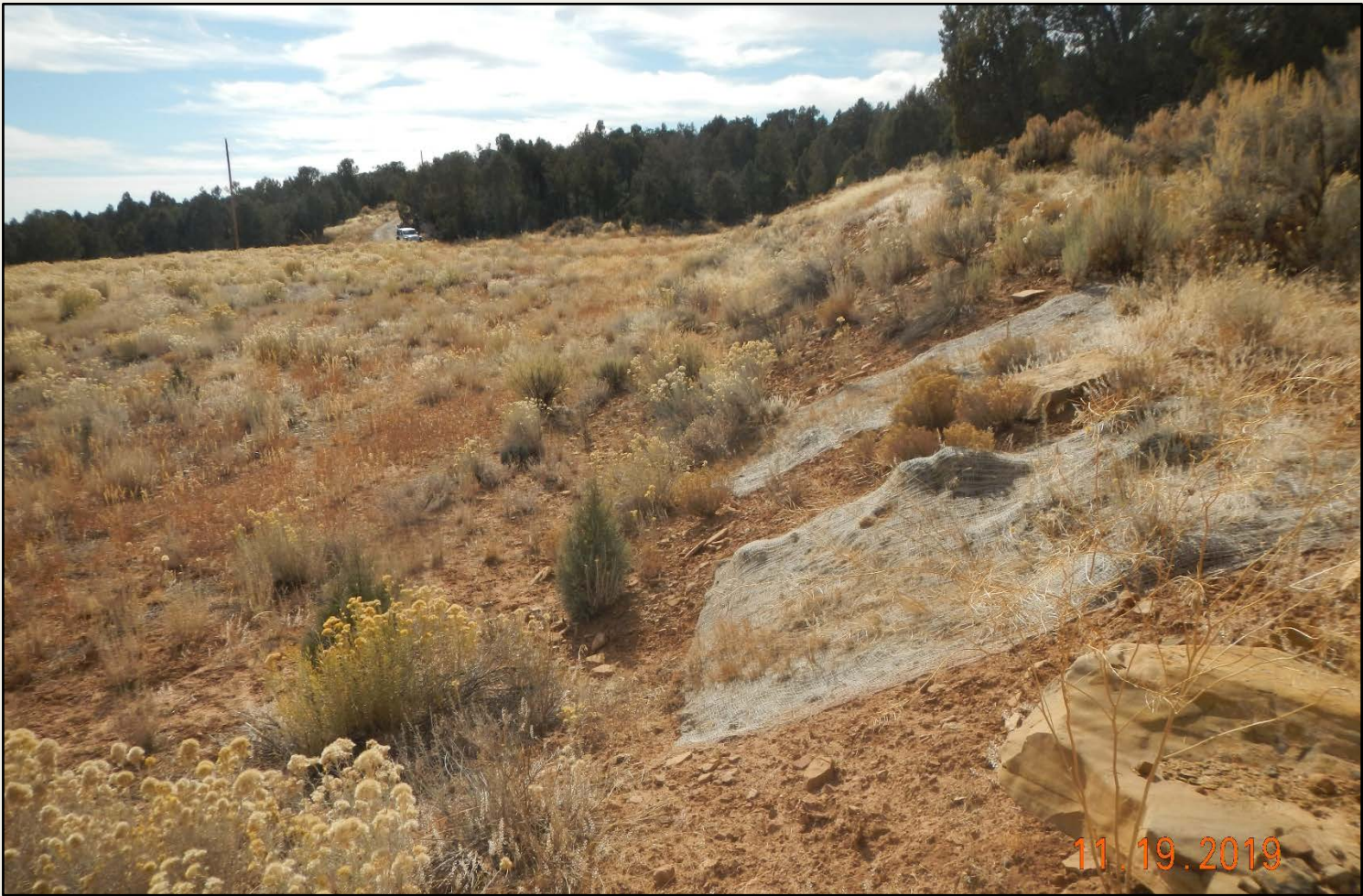
Photo 3. View of the western project from northwestern corner facing southward. Erosion blankets are in place on portions of the cut-slope, but portions of the cut-slope remain bare.
