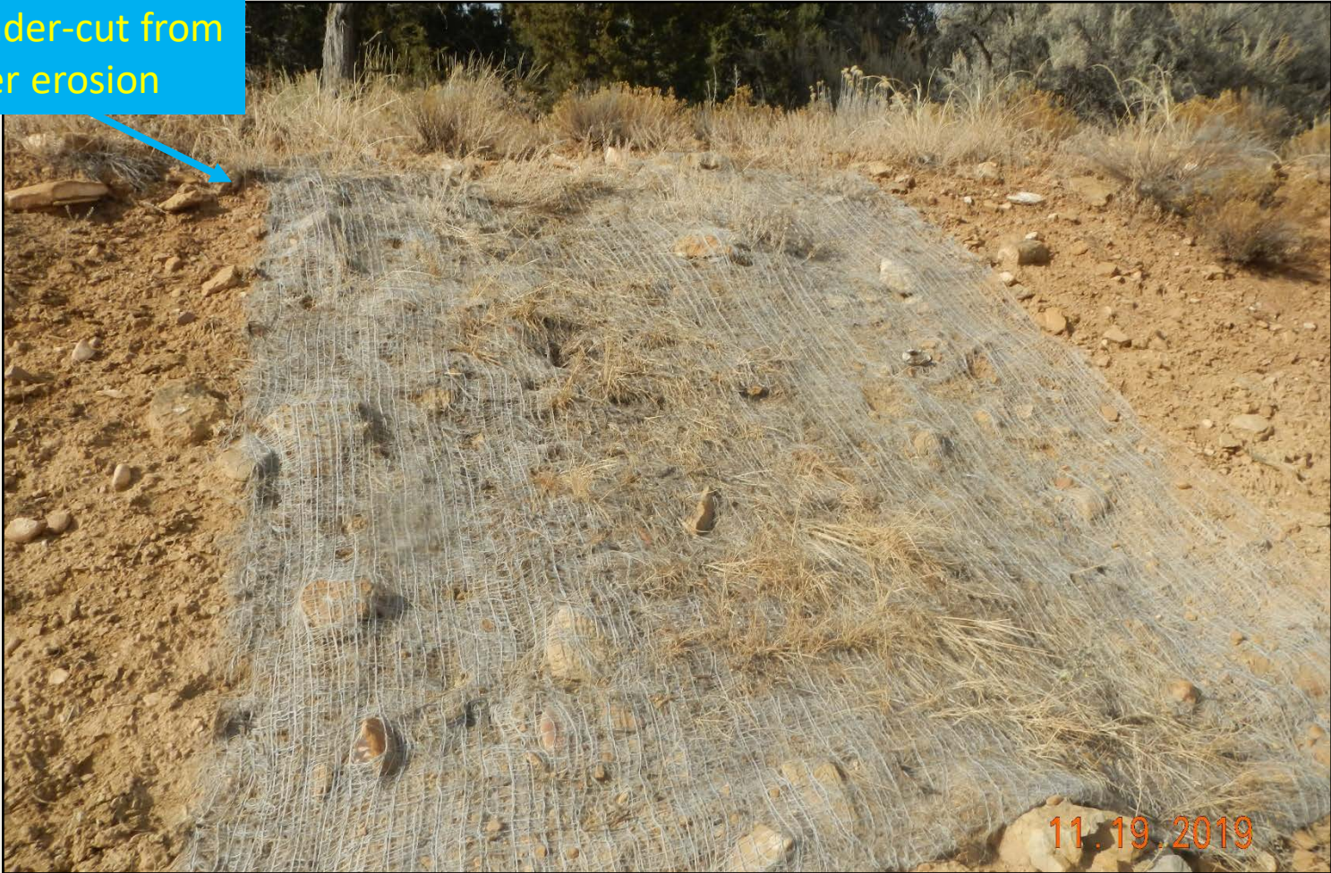
Photo 4. Closeup view of erosion blanket on the western cut-slope. Perennial vegetation is becoming established in the center of the blanket, but not on outer edges or on bare soils that remain on the cut-slope. Vegetation at top of slope is under-cut by erosional processes. Vegetation at top of slope is under-cut from stormwater erosion.
