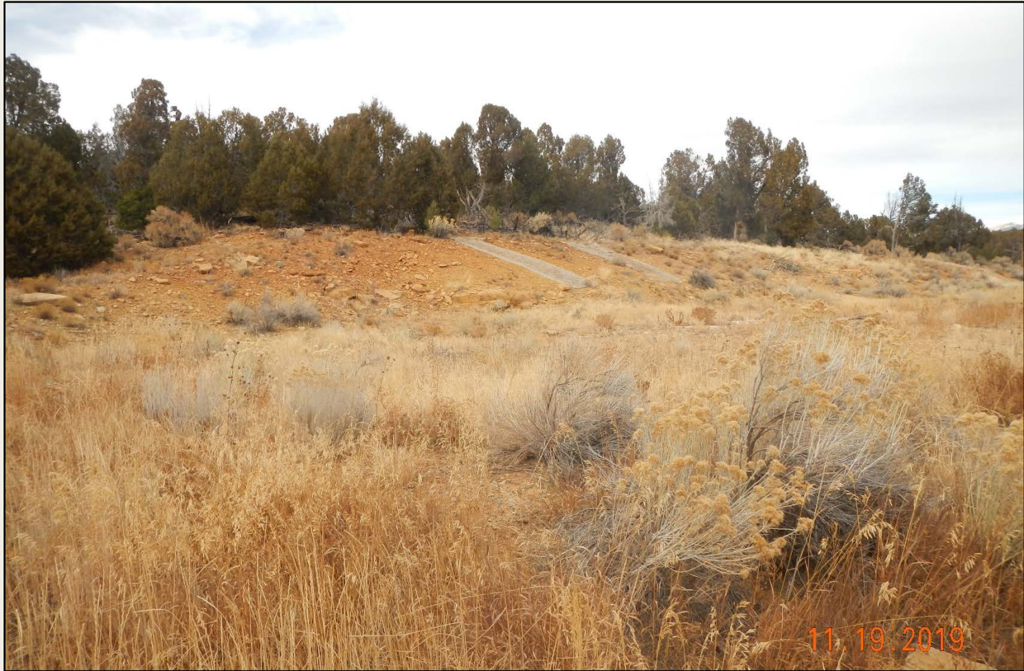
Photo 2. View of the southwestern cut-slope from the well pad entrance. Bare soils on well pad cut-slope remain unstabilized. Erosion blankets and seeding should be conducted across the southwestern slope, not just in the 2 small areas shown.
