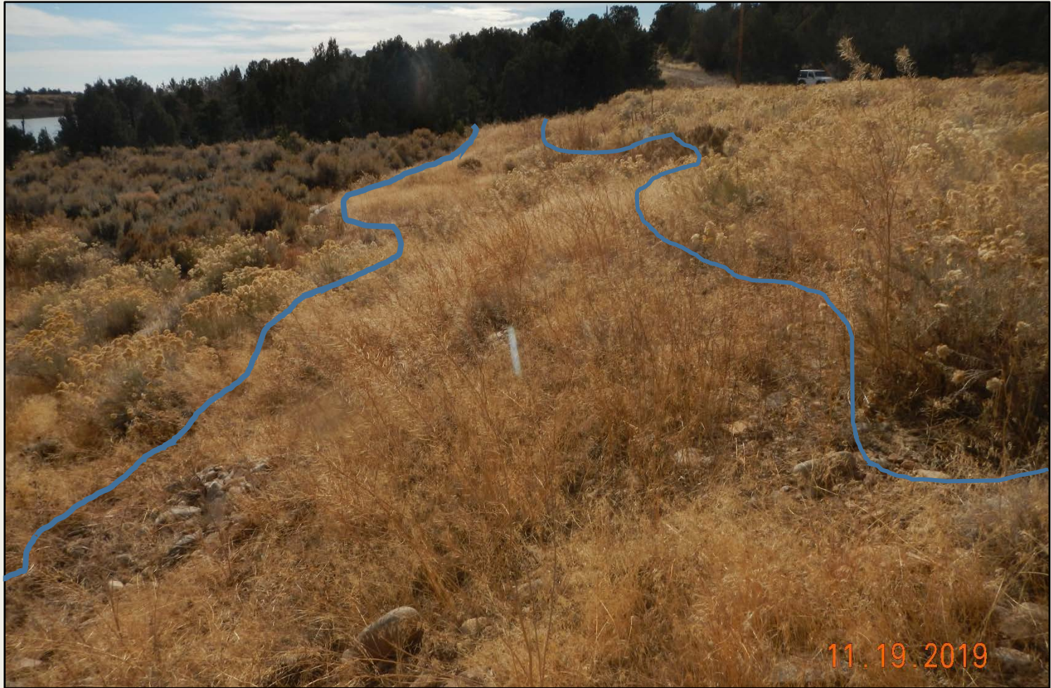
Photo 6. View of the eastern fill-slope facing southward. Vegetation between the two blue lines is largely annual species and not stabilized with desirable perennial vegetation.
