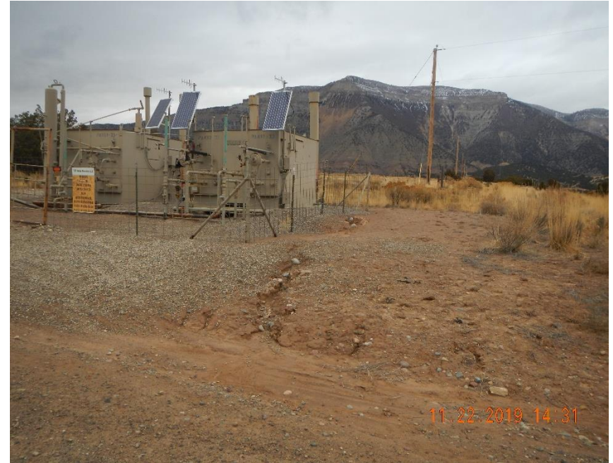
Sediment washing from around separators into roadside ditch.
