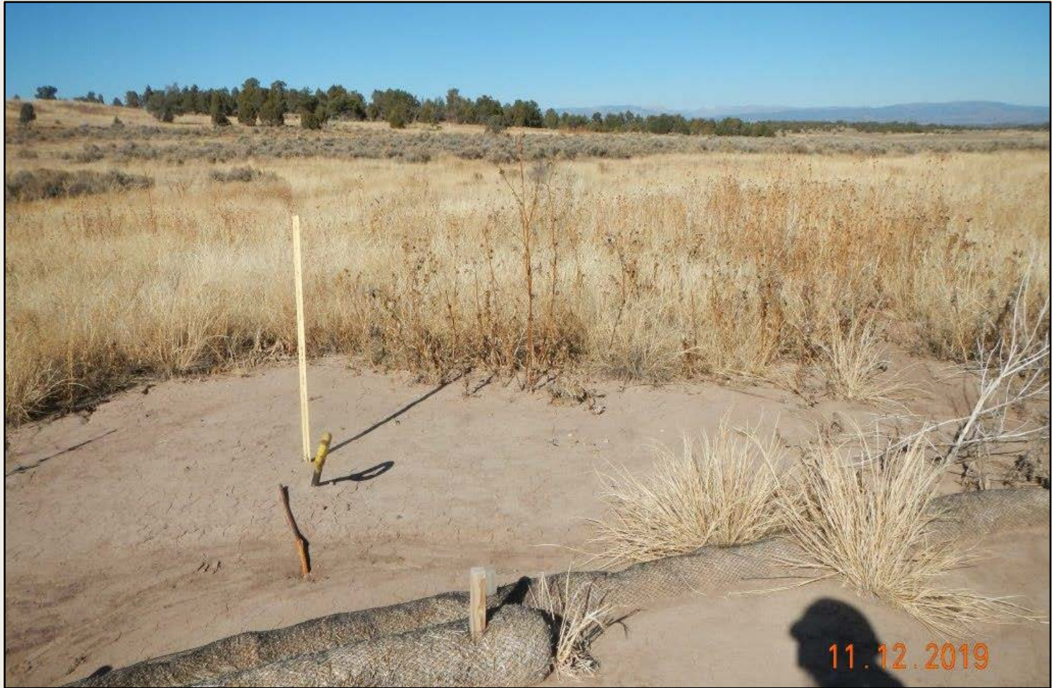
Photo 3. View of sediment deposition and wattles filling with sediment, downslope of erosional channels in Photo 2. Sediment flows off of the working area in this corner.
