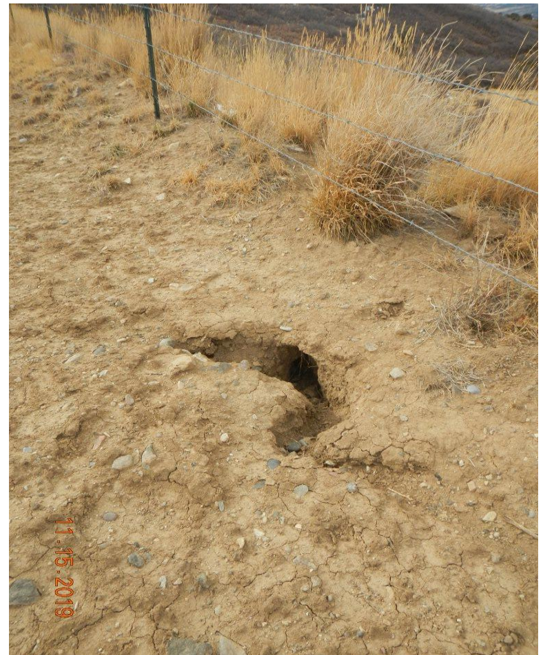
Photo#3: Subsidence, worm hole on Northwest edge of Pad.
