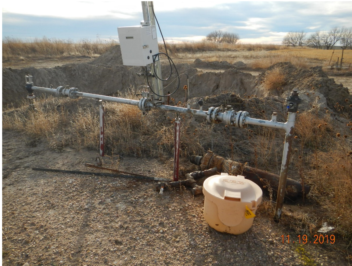
Photo # 9 – Unused equipment and flowline risers need to be removed
