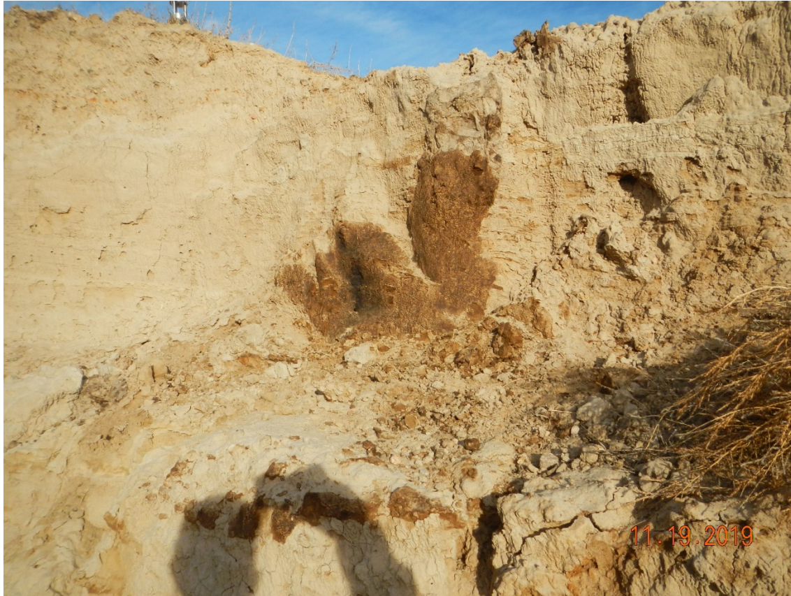
Photo # 8 – Petroleum impacted soil remains in the east wall of the pit excavation
