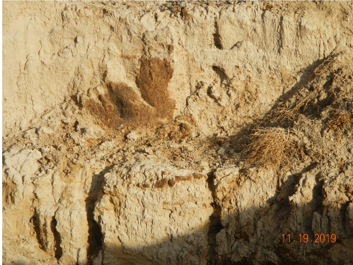
Photo # 3 – View east at east wall of pit excavation, oily soil requires removal
