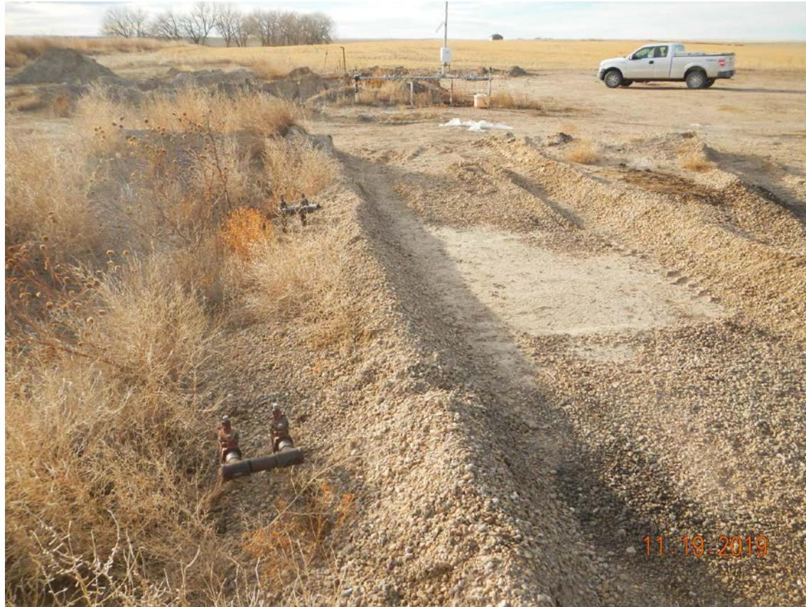
Photo # 10 – View west from former tank battery area, flowline risers, gravel require removal
