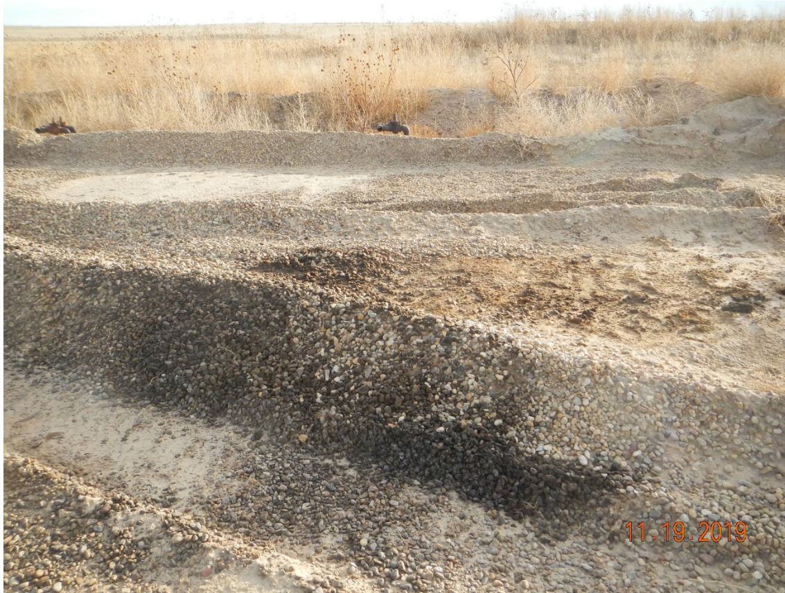
Photo # 11 – View south at former tank battery area, flowline risers, oily gravel require removal
