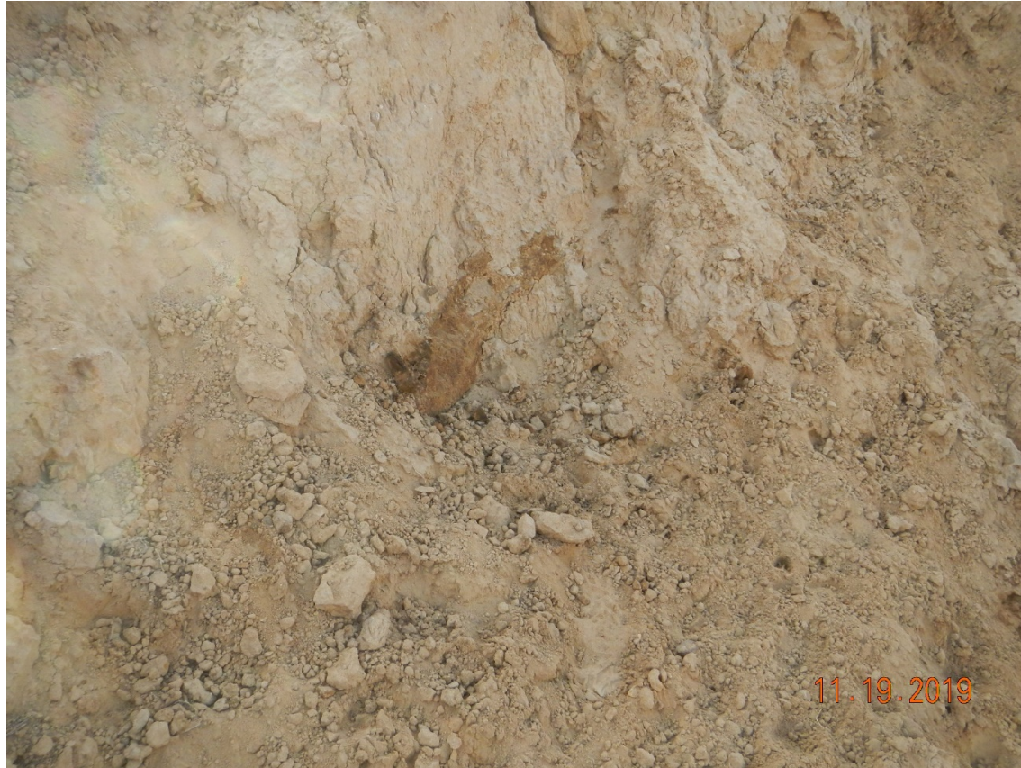
Photo # 6 – Petroleum impacted soil remains in the southwest wall of the pit excavation
