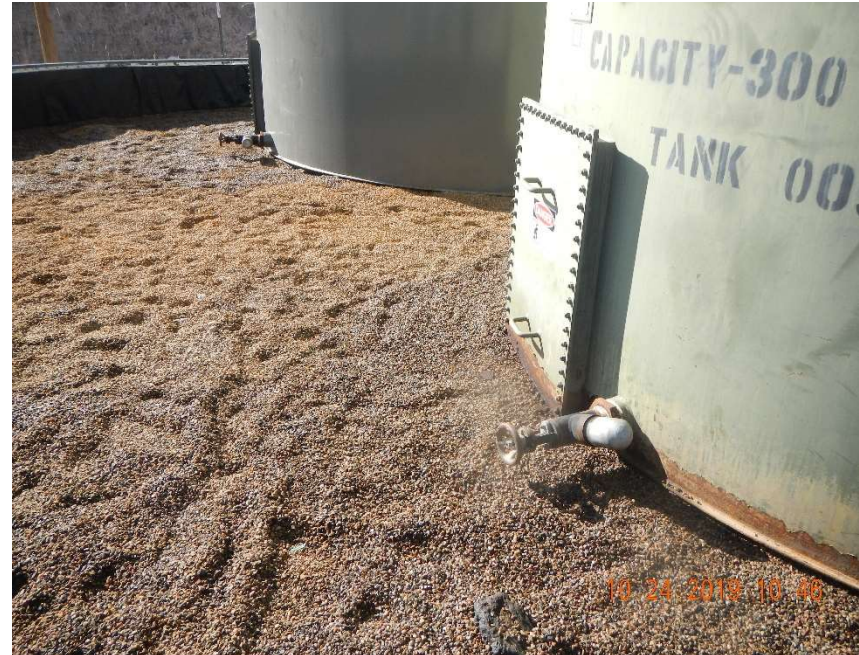
Photo #14 - View of the impacted gravel in the eastern section of the tank battery.
