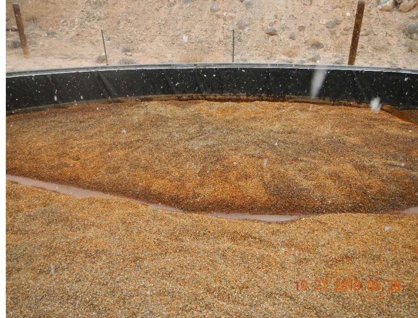
Photo #4 – View of the residual staining ring approximately three to four inches above the gravel in the tank battery.
