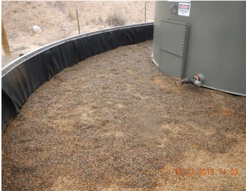
Photo #7 – View of the impacted gravel in the eastern section of the tank battery.
