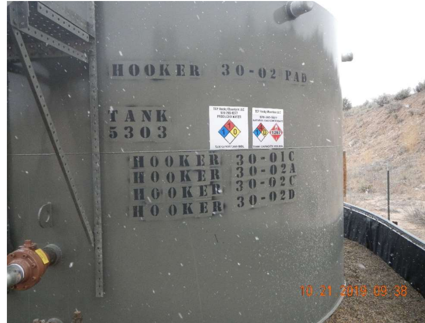
Photo #6 – View of the replacement 300 BBL Condensate and Produced Water AST.
