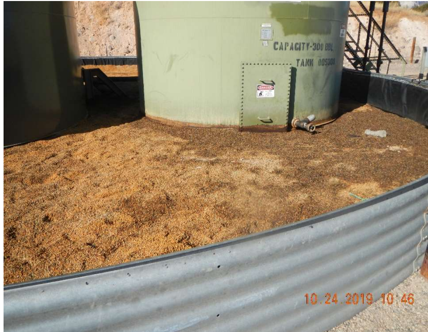
Photo #15 - View of the impacted gravel in the eastern section of the tank battery.
