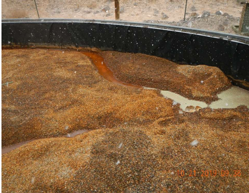
Photo #1 – View of impacted fluids on the west side of the tank battery.
