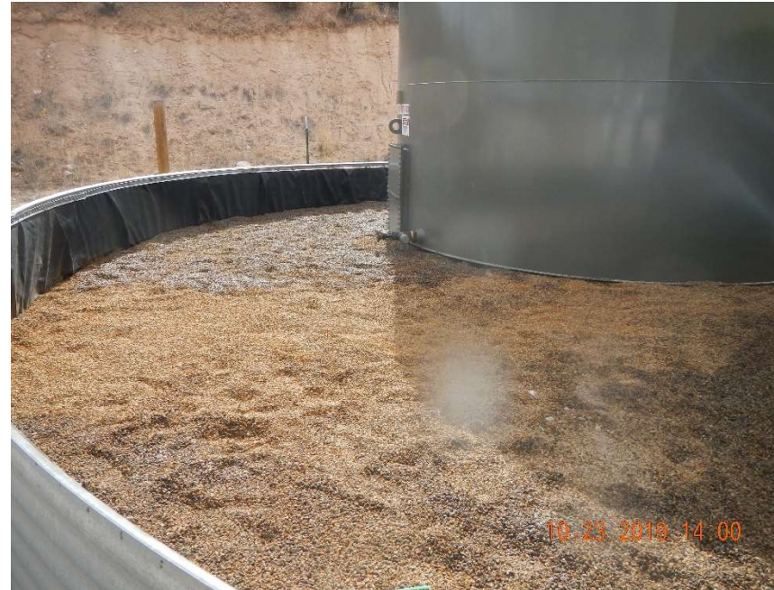
Photo #8 - View of the impacted gravel in the eastern section of the tank battery.
