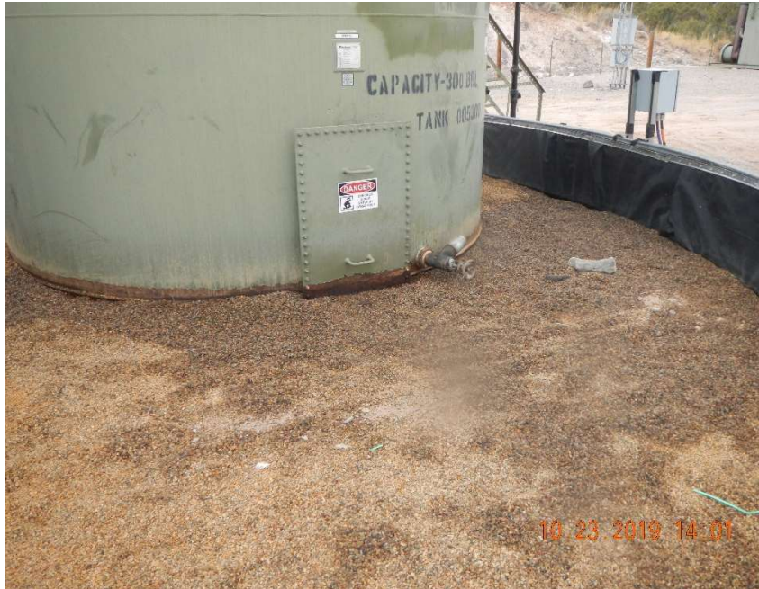
Photo #9 - View of the impacted gravel in the eastern section of the tank battery.
