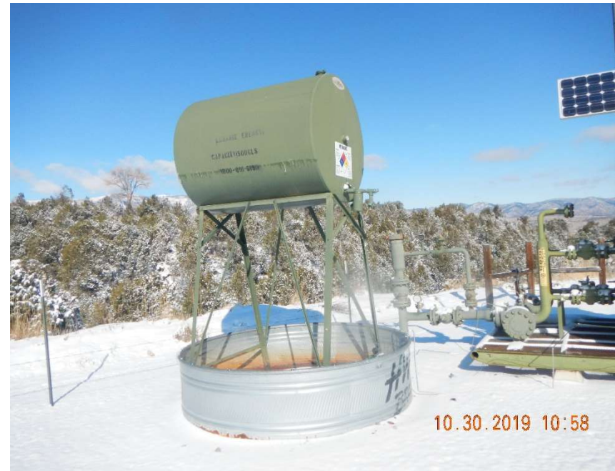
Photo #20 – 500 Gallon Methanol Tank labeled Laramie Energy.
