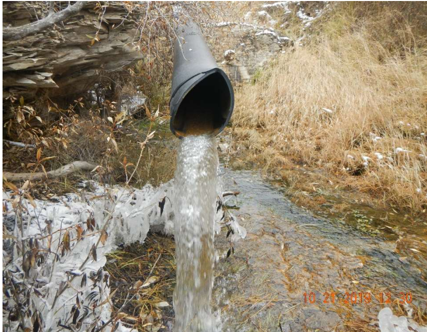
Photo #5 – View of the ruptured poly pipe.
