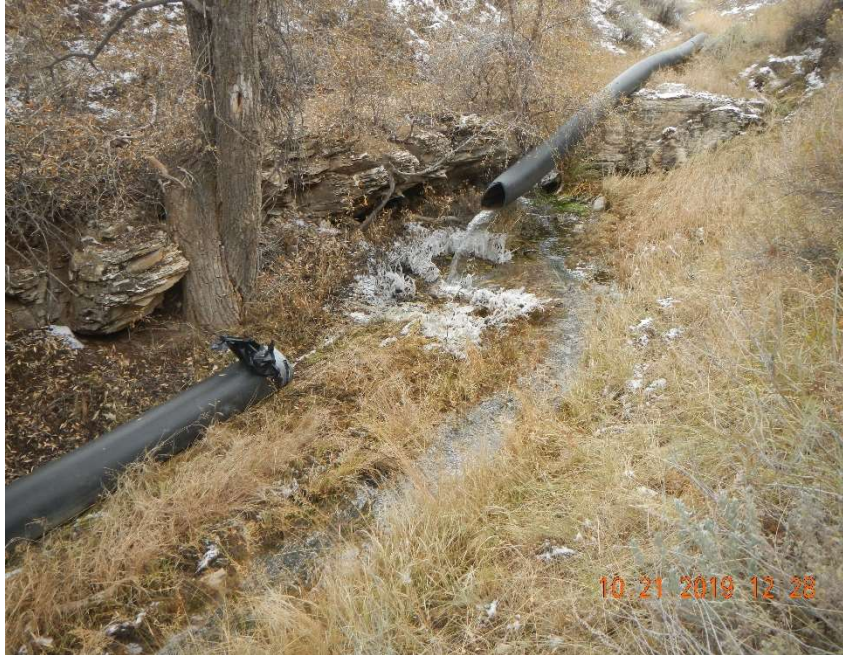
Photo #3 - View of the ruptured poly pipe looking south.
