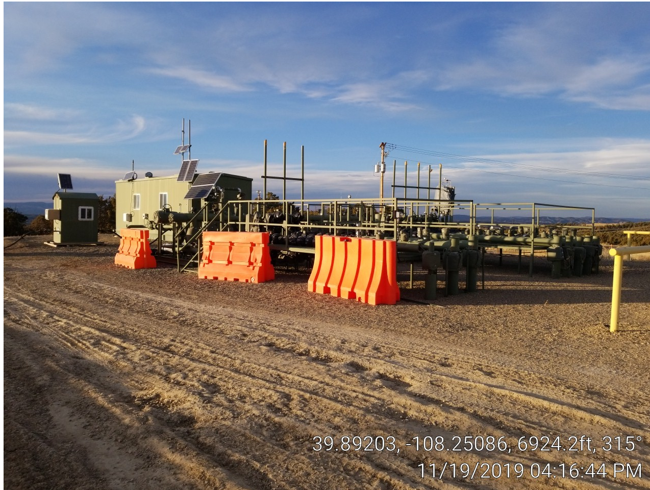
Photo 2. Separator & well header.
