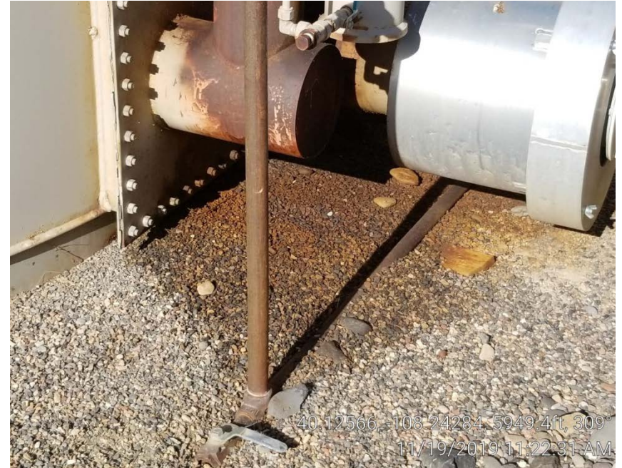
Photo 3. Stained gravel at tank.
