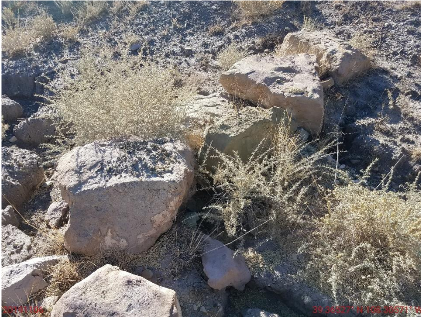
Photo 9: Photo taken from the location. Photo shows what appears to be a rock-check installed in the low areas of the location. BMP does not appear to have been constructed in accordance with good engineering practices and is not in proper functioning condition.
