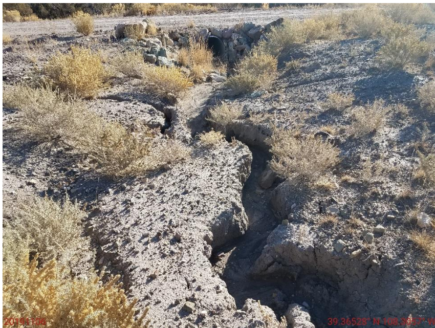
Photo 11: Photo of culvert under access road and erosion degradation.
