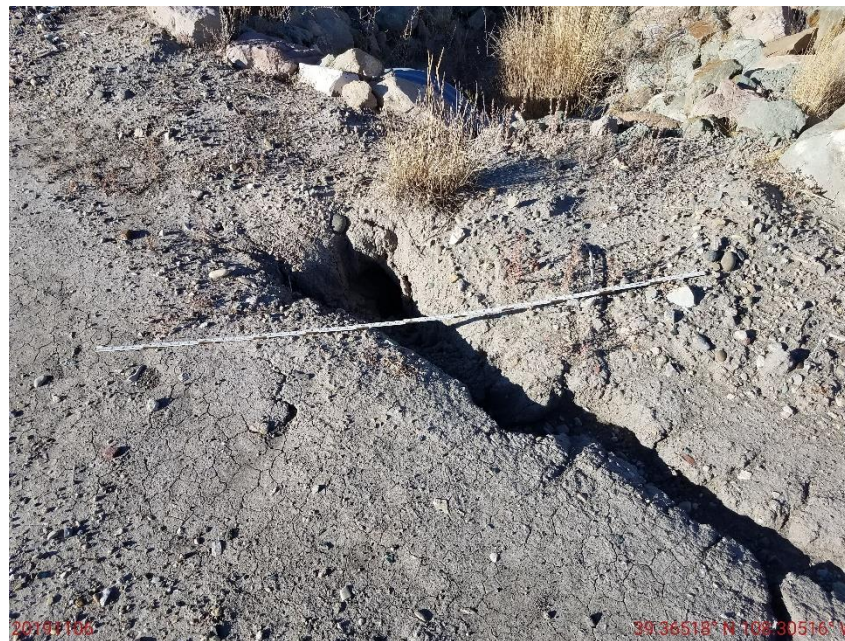
Photo 2: Photo taken from the culvert adjacent to the access road. Photo shows stormwater erosion degradation. 6 foot measuring stick for reference area.
