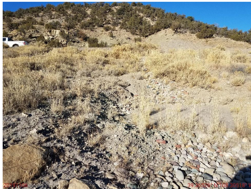
Photo 12: Photo taken down-slope of the culvert. Photo shows erosion degradation due to stormwater runoff from the location.
