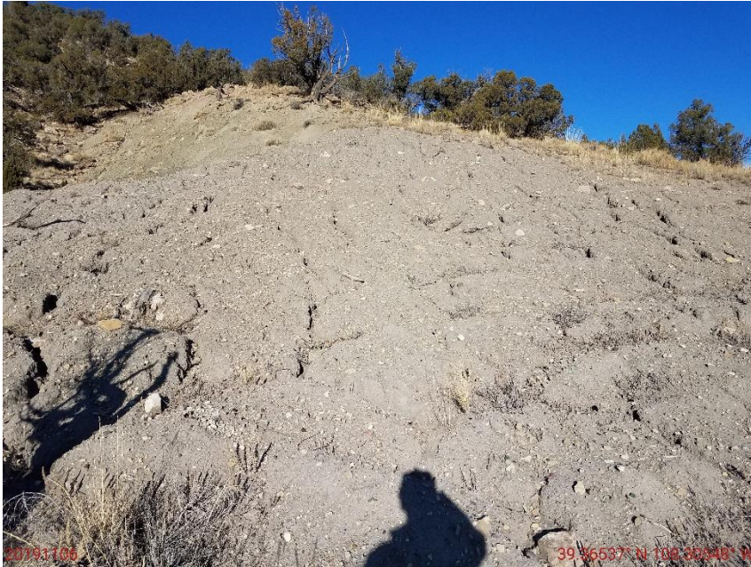
Photo 3: Photo taken from the location, facing west. Photo shows stormwater erosion degradation occurring throughout location. Operator has failed to conduct ongoing stormwater monitoring and management, resulting in reclamation failure of the location.
