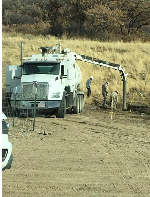
**Hydrovac truck on location digging down to flowline.**
